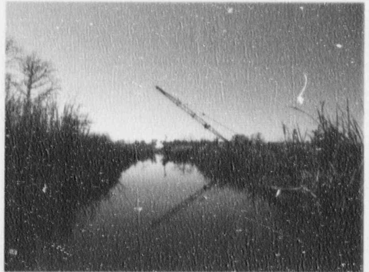
Underwater cables deliver power to Waccamaw Neck region with minimal disturbance to the environment.
