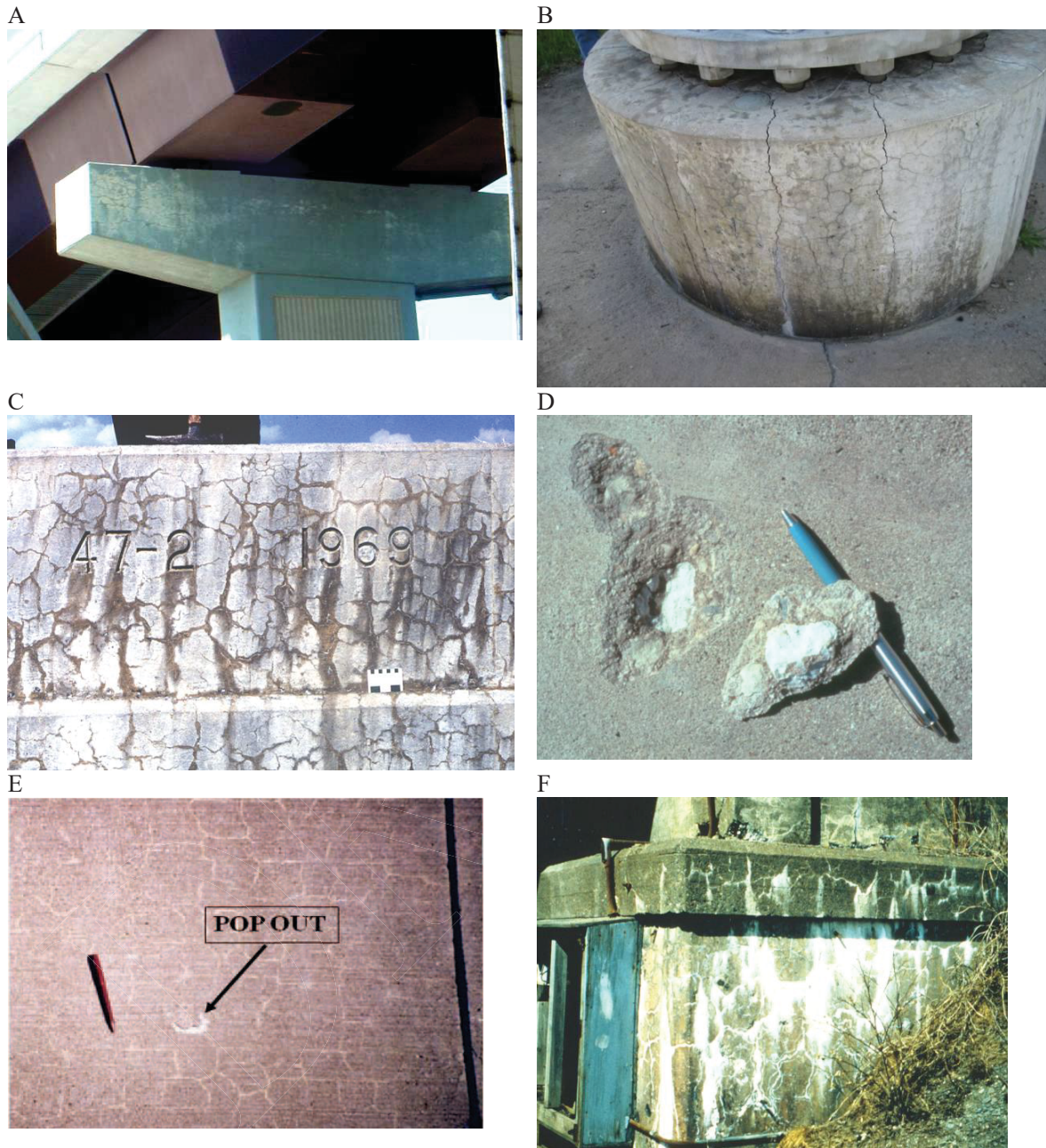
Figure A2. (A). Bent cap in relatively new bridge structure showing signs of ASR, primarily where direct access to moisture/rain prevails. (B). ASR cracking in drilled shaft supporting high-mast illumination pole. (C). Gel staining around cracks in the parapet wall of a bridge structure affected by ASR. (D). Pop-out created by the expansion of a frost-susceptible porous coarse aggregate particle. (E). ASR-induced pop-out in a concrete pavement incorporating highly-reactive aggregates; also noted pattern cracking (F). Efflorescence and exudations of alkali-silica gel at the surface of the concrete foundation of 25-year-old highway bridge affected by ASR.
