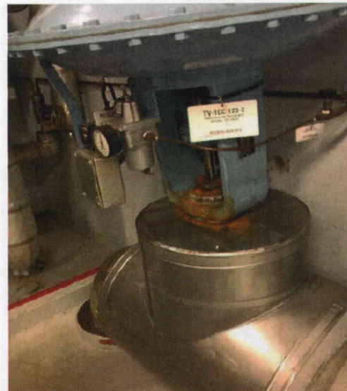
Figure 6-2: Corroded valves with old deficiency tags.
