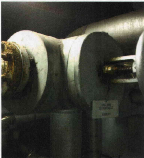
Figure 6-2: Corroded valves with old deficiency tags.
