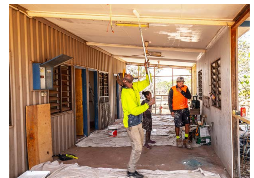
Maurice Simon Jr applies new paint at Marralum.
