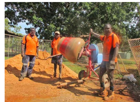
Locals working on a remote housing site in Weemo.
