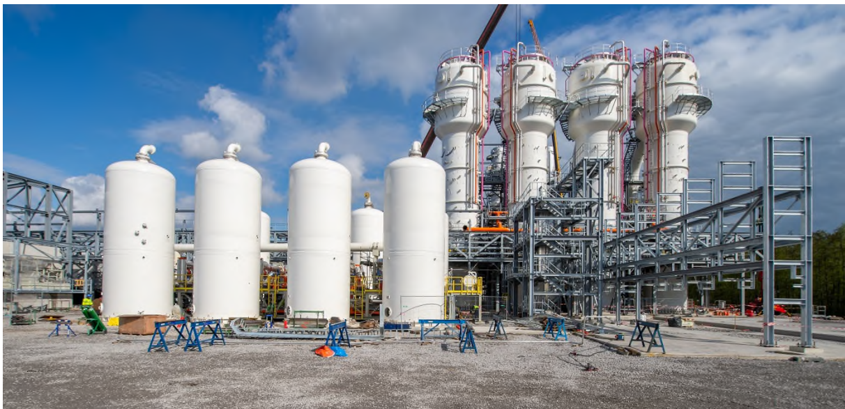
Figure 100: Steelanol plant under construction at ArcelorMittal Gent
