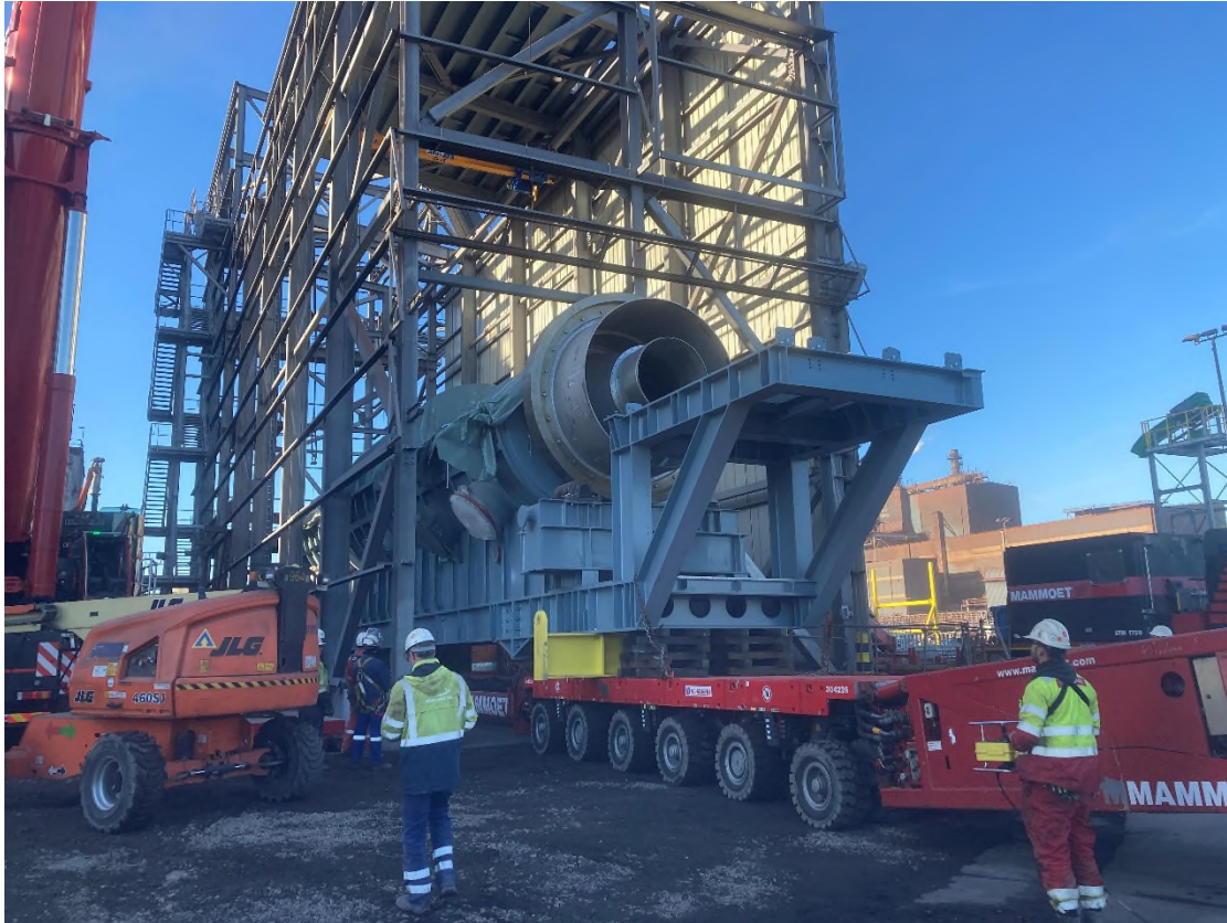
Figure 95: Rotating Drum installation in February 2022
