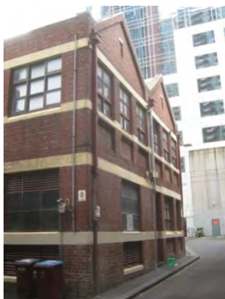
Figure 4. 1-3 Evans Lane, constructed in 1913.
