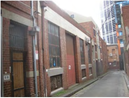
Figure 6. 12-14 Guildford Lane, constructed c 1920.
