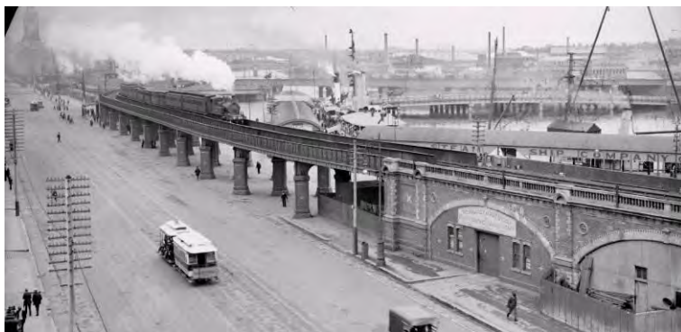
Figure 4. Extract from a c1911 photograph showing the double-line viaduct with a steam locomotive running on it. The viaduct buildings can be seen on the right-hand side. (Source: 'Looking east along Flinders Street', c1911, SLV)
