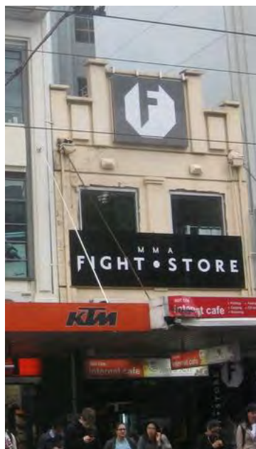
Figure 10. 349 Elizabeth Street, built in c1920s.
