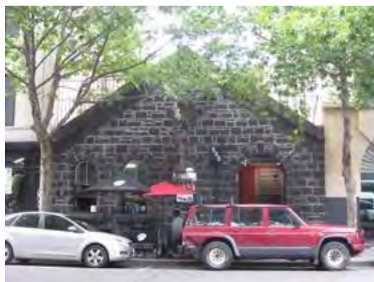
Figure 10. 585 Little Collins Street constructed 1865.
