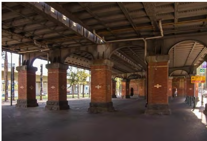
Figure 13. View towards west, near intersection of William and Flinders streets. Three piers on the left-hand side are from 1891 and one on the right-hand side is from 1917. (Source: Context 2019)
