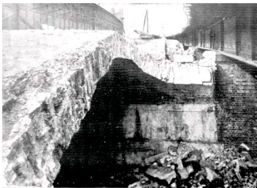
Figure 7. The arches near the Fish Market were demolished in 1916 and replaced with iron girders. ( Australasian 23 September 1916:54)
