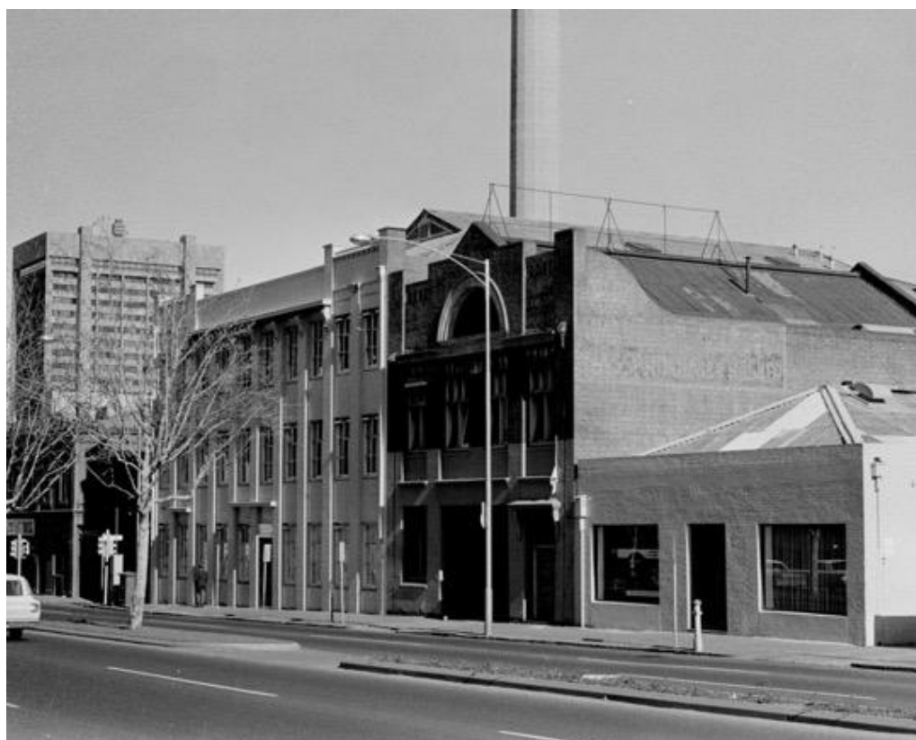
Figure 4. A 1960s photograph of King Street West between Little Lonsdale Street and Nicholson Place, showing 295-305 King Street. (Source: Halla c1960-1969, SLV)
