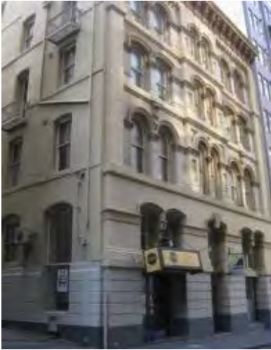
Figure 3. 392-396 Little Collins Street constructed 1882-3.
