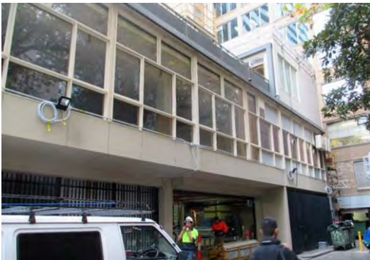
Figure 8. 2-18 Ridgway Place, built in 1958. (Source: Context, 2017)
