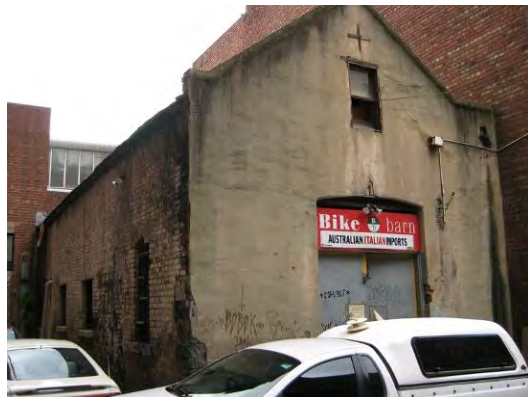
Figure 9. Rear of 361 Little Lonsdale constructed 1854.
