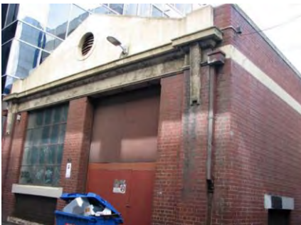
Figure 8. Substation, 10-14 Park Street constructed 1928. (Source: Context 2017)
