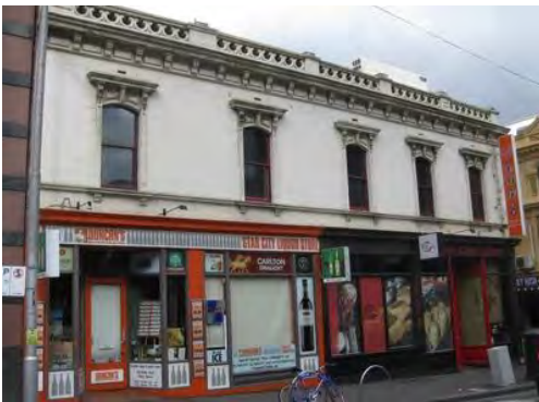
Figure 11. 189-195 Exhibition Street, built in 1882. (Source: Butler 2011)
