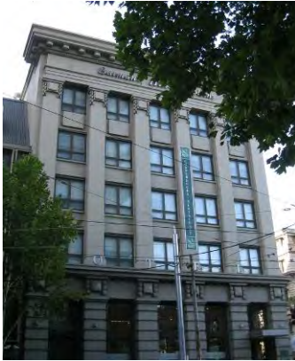
Figure 2. 615-623 Collins Street constructed 1923-24.
