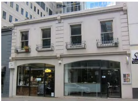
Figure 9. 470-472 Little Lonsdale Street, built in 1872. (Source Context 2017)
