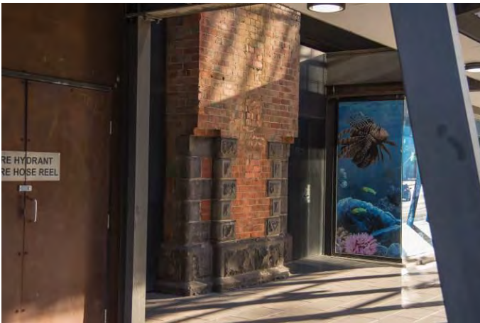
Figure 15. One of the piers partially retained, now incorporated into the shell of the aquarium. (Source: Context 2019)
