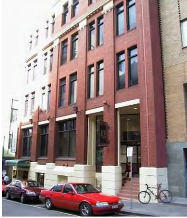
Figure 9. 401-405 Little Bourke Street, built in 1911.
