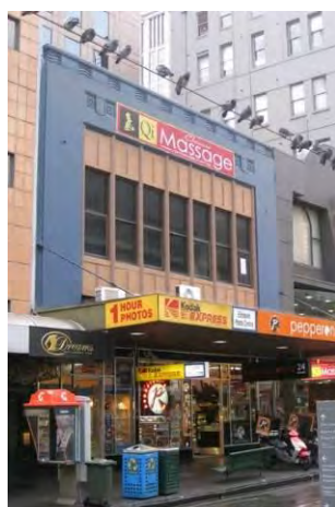
Figure 4. 7-9 Elizabeth Street, constructed in 1933.
