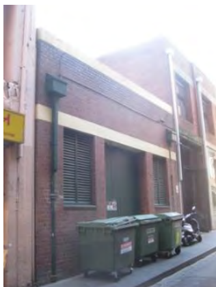
Figure 5. 28 Crossley Street, construction date unknown.
