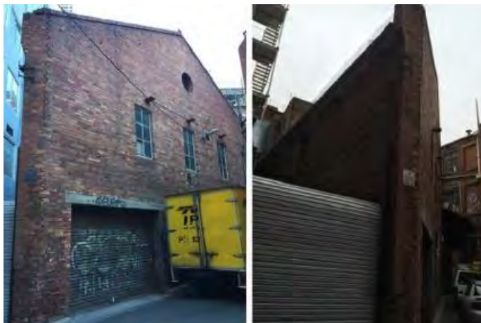
Figure 5. Rear of 369-71 Lonsdale Street constructed 1888.
