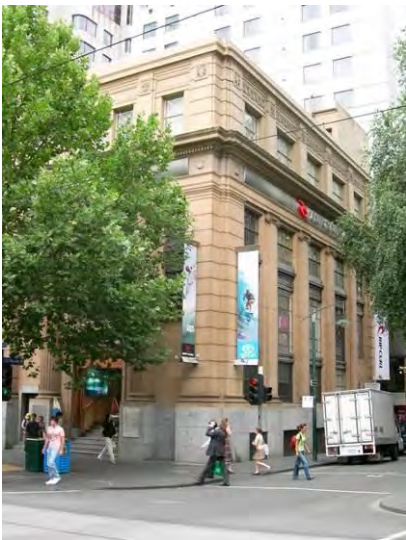
Figure 12. 119-225 Swanston Street, built in 1928 (Source: VHD)
