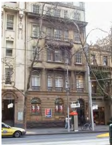
Figure 5. 10-12 Collins Street built in 1916-1925.
