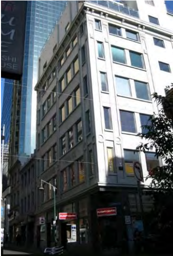
Figure 5. 386-392 Little Bourke Street, built in 1926.
