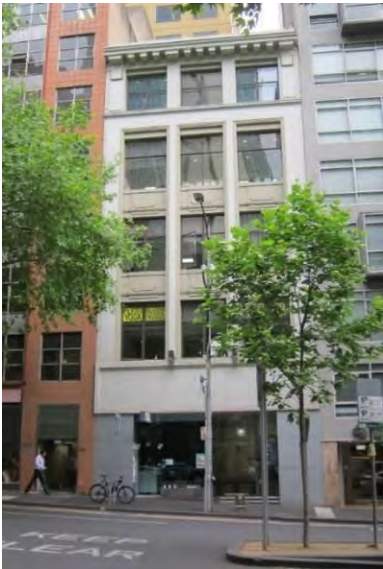
Figure 9. 410-412 Lonsdale Street, built in 1922. (Source: Context 2018)
