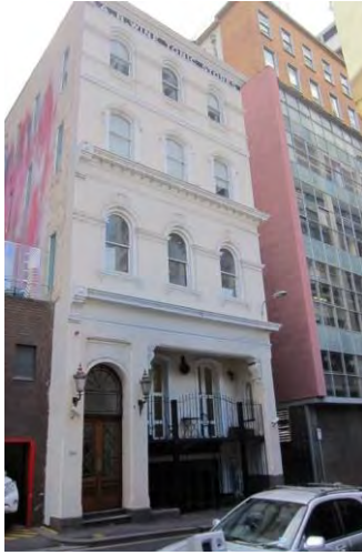
Figure 9. 384-386 Flinders Lane constructed 1885 and 1888. (Source: Context 2018)
