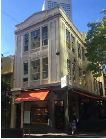
Figure 8. 386-392 Little Bourke Street, built in 1926.
