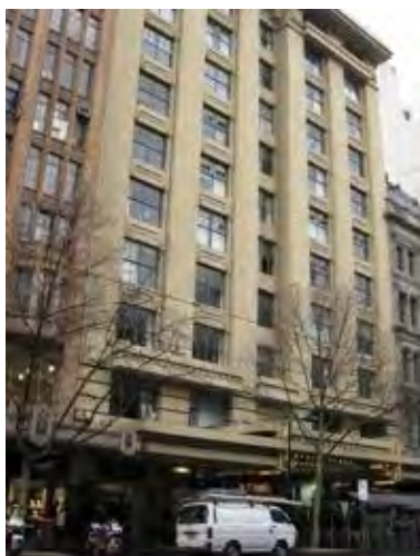
Figure 3. Capitol Arcade, 115 Swanston Street constructed 1924.
