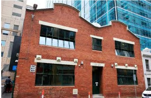
Figure 6. 27-29 Little Lonsdale Street, constructed in 1924.
