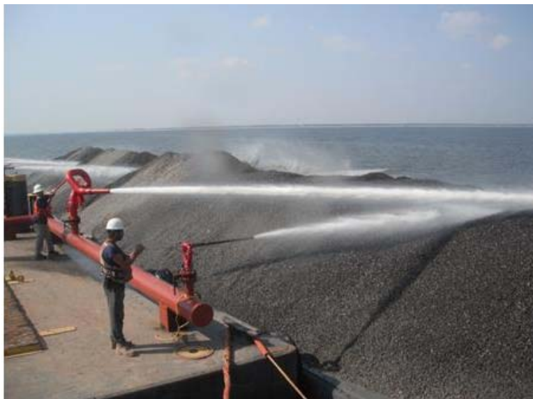
Oyster cultch being deployed in the fall of 2012.
