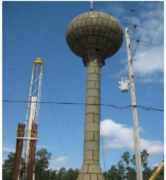
Stone County Ten Mile Road water project
