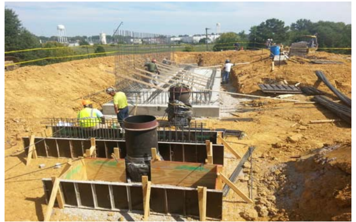
City of West Point Wastewater Treatment Plant Project
