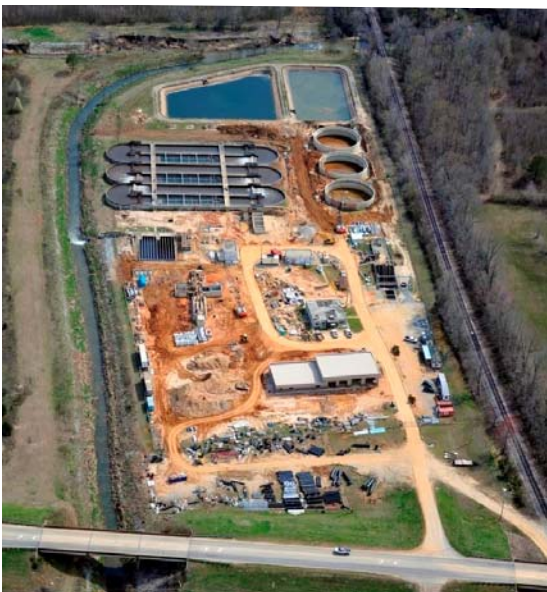
City of Corinth Wastewater Treatment Plant
