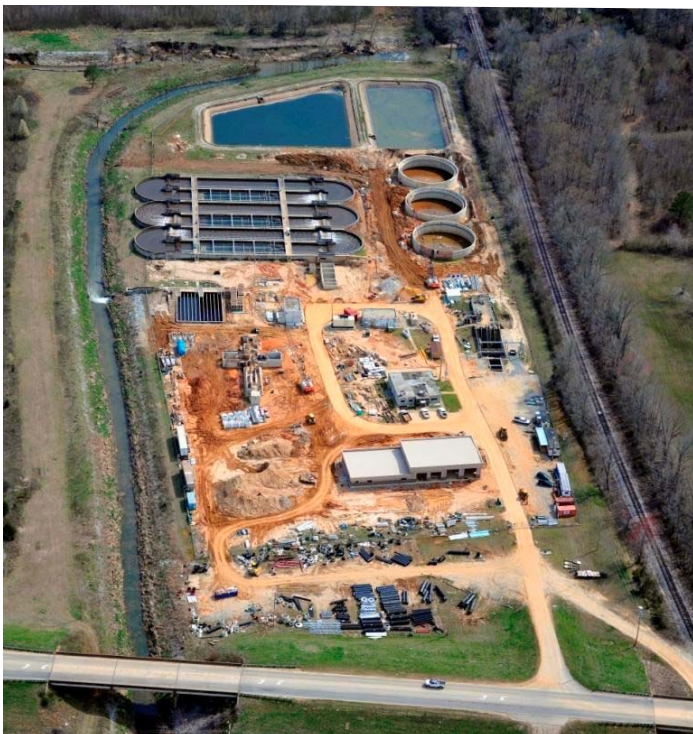
City of Corinth Wastewater Treatment Plant Project
