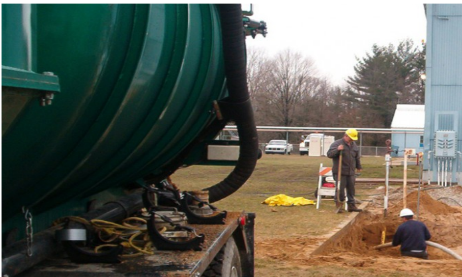
Vacuum Truck Cleanup at a UST Site
