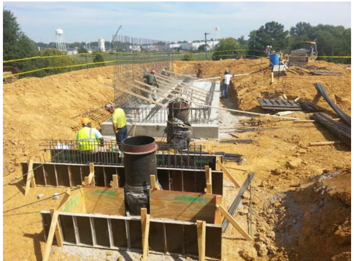
City of West Point Wastewater Treatment Plant Project
