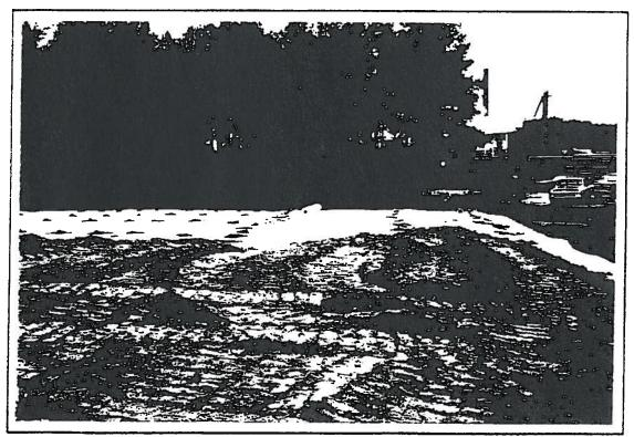
PHOTO 20: Placing Filter Fabric onto Drainage Layer and Pushing Cover Soil onto the Fabric
