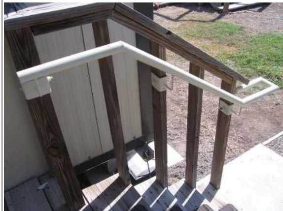
Photo #27: Re-paint all metal pipe handrails
