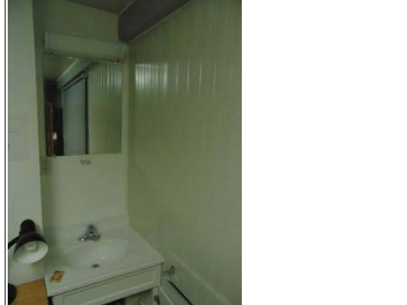
Photo #58: Typical sink/cabinet assembly
