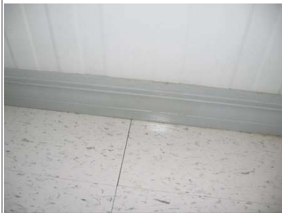
Photo #15: Typical painted wood baseboards
