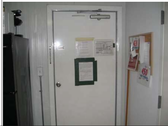
Photo #14: Typical solid metal exterior door and frame
