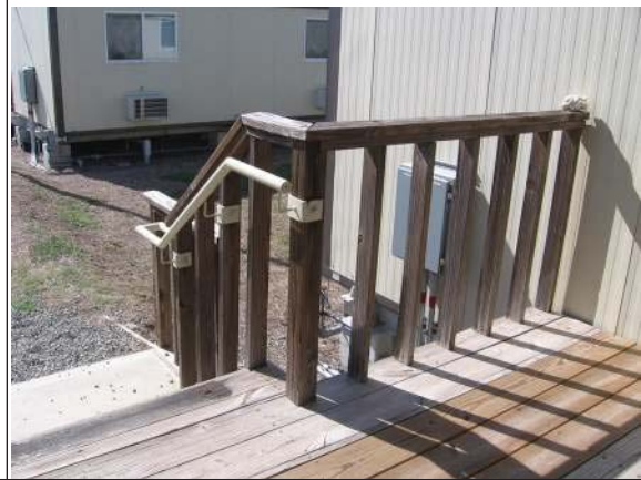
Photo #276: Typical pressure treated wood railing
