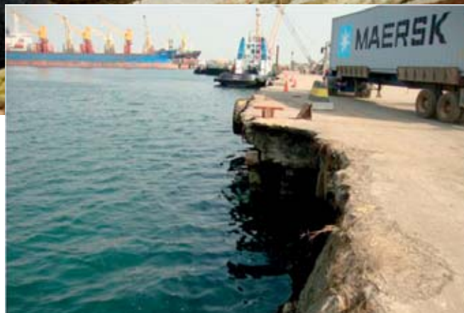
APM Terminals expects to invest USD 120 million in the port over the course of the 25-year concession.
