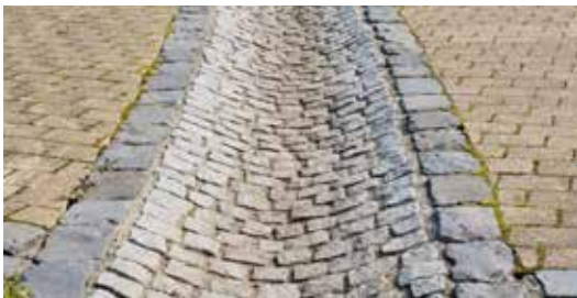
Sidewalk runnels would visibly convey water from impervious surfaces to the raingardens.
