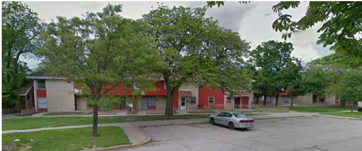
Photo from Google Street View
