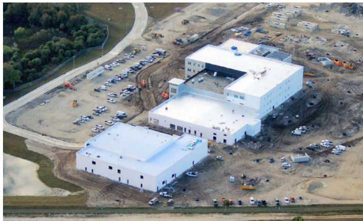
Construction of Gateway High School Source: SDLC
