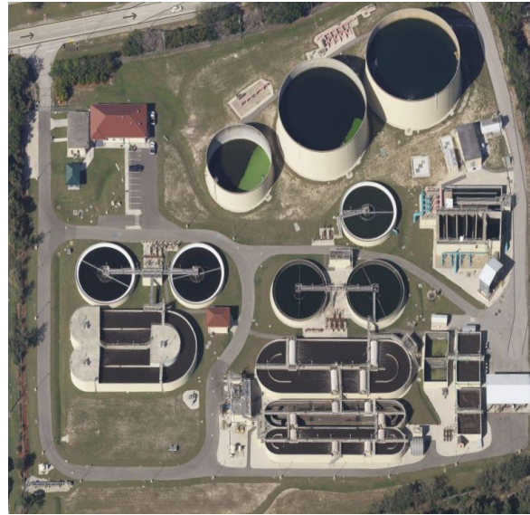
Three Oaks Water Reclamation Facility Source: Lee County Utilities
