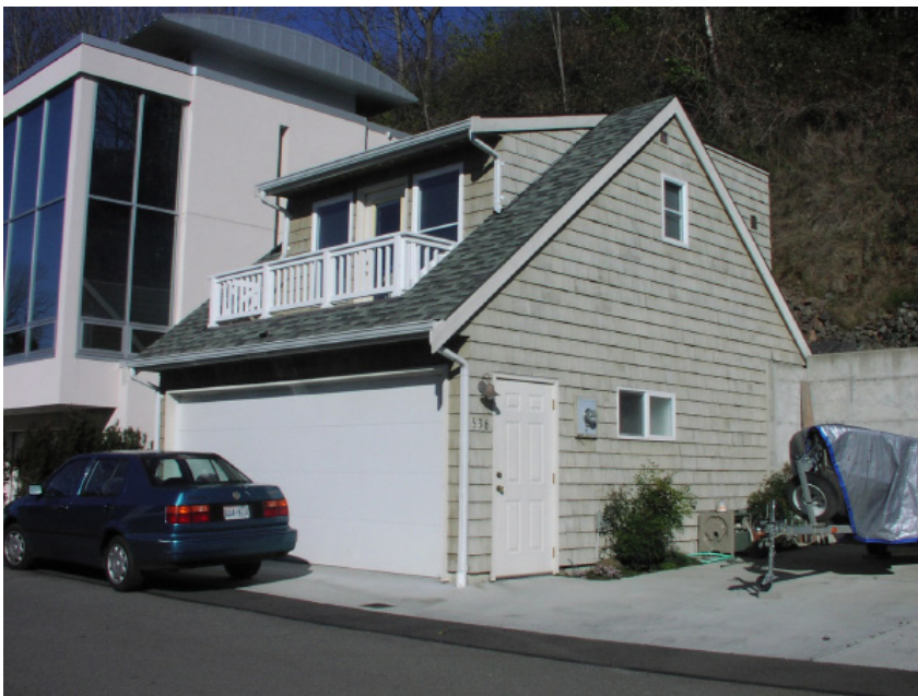
Example of an ADU in Kirkland above a detached garage
