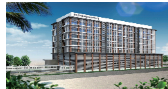
Philippine Railway Institute (Under construction)
