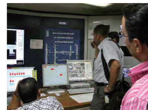
Scene from tour of Otemachi Station Disaster Prevention Control Office
