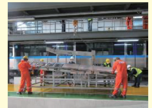
Removing air-conditioning unit from car body
