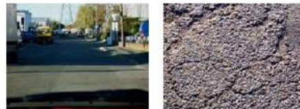
Cobblestone Road (vehicle speed 30 Km/h)
