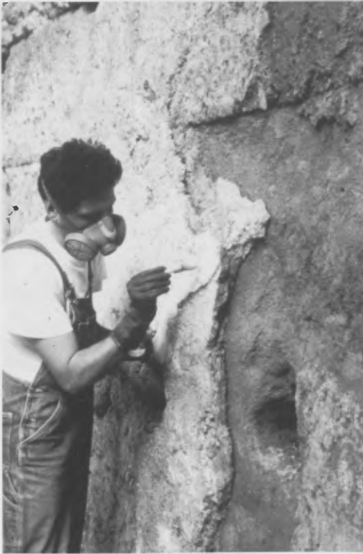
Figure 1. Plaster on tuff: application of tissue for temporary consolidation of perimeter strip. Photo: author.
