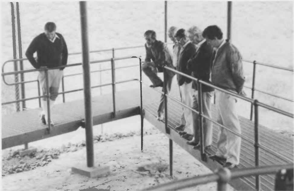
Figure 7. Visitors on the walkway. Note the roof columns and walkway supports embedded in the surface.
