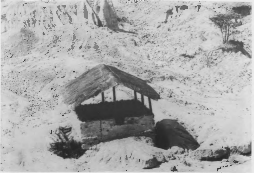
Figure 6. On-the-spot museum - a poorly built shelter that causes decay of fossil fauna, mainly in rainy seasons.
