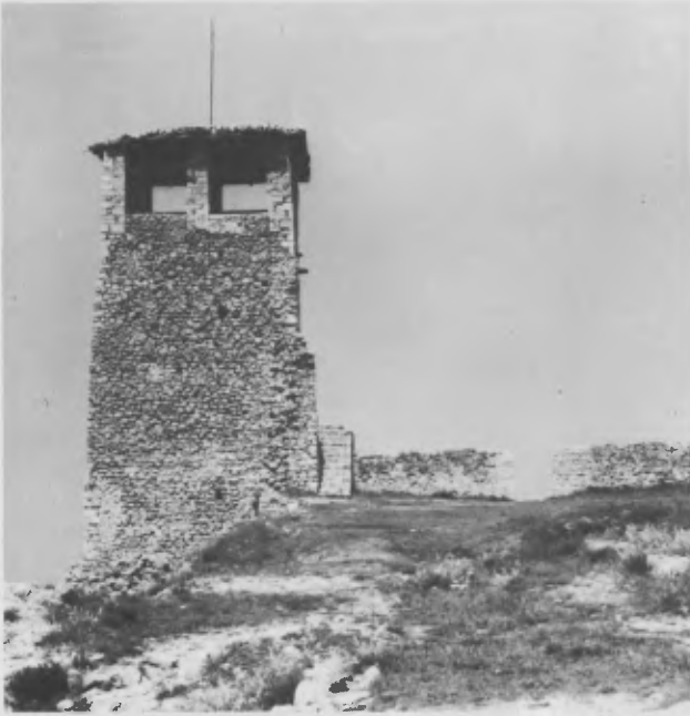
Figure 7. The acropolis of the castle: prior to excavation.
