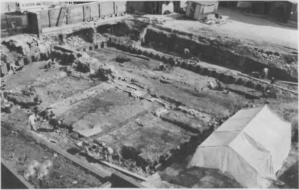
Figure 2. The excavation site at Billingsgate, City of London, in 1982, after the clearance of modern basements and insertion of sheet piling to define an area 20x25 m. The excavation thereafter lasted one year and excavated this area down to a depth of 6 m (Museum of London).
