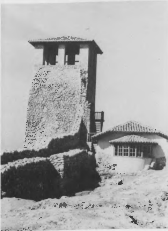
Figure 17. Acropolis: the definitive conservation of the southern tower.
