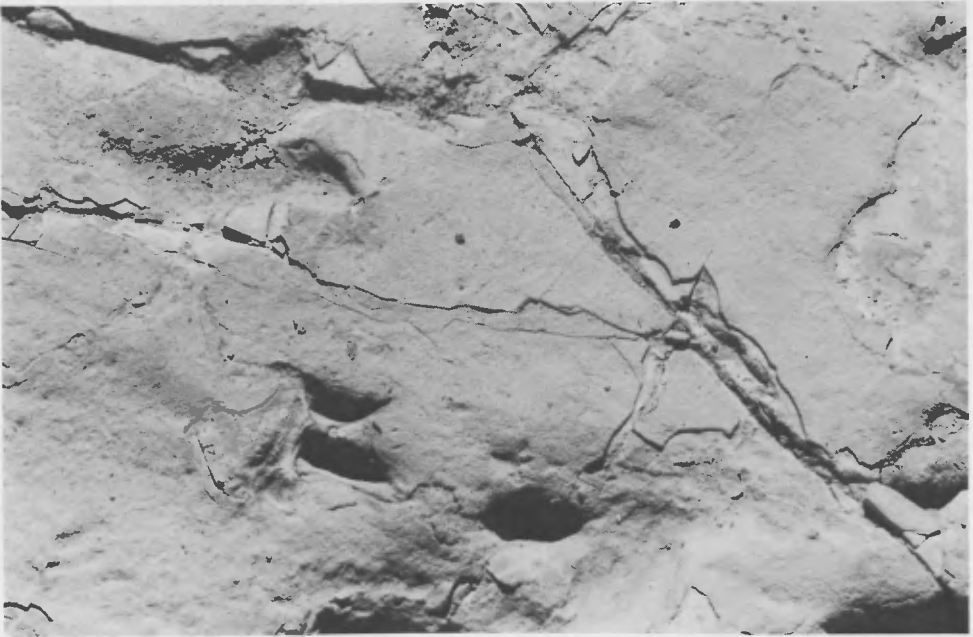
Figure 6. Cracks in the surface and lifting of the thin limonite layer.
