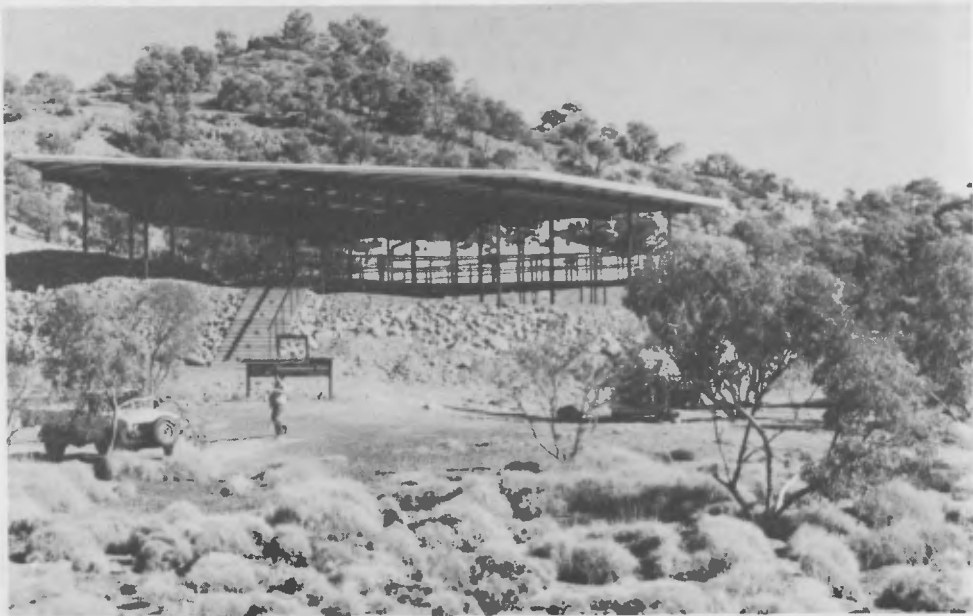
Figure 5. Roof, walkways and fence around the site. Scree slopes were formed from overburden of sandstone excavated to uncover the tracks.
