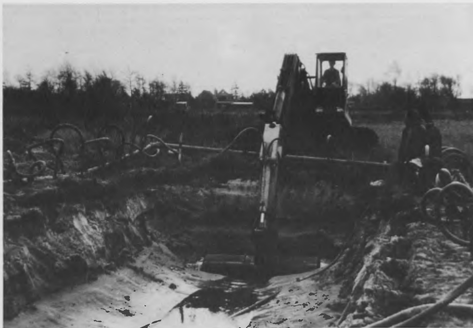
Figure 4. The suction-tube system along the edges of the deposition pit.
