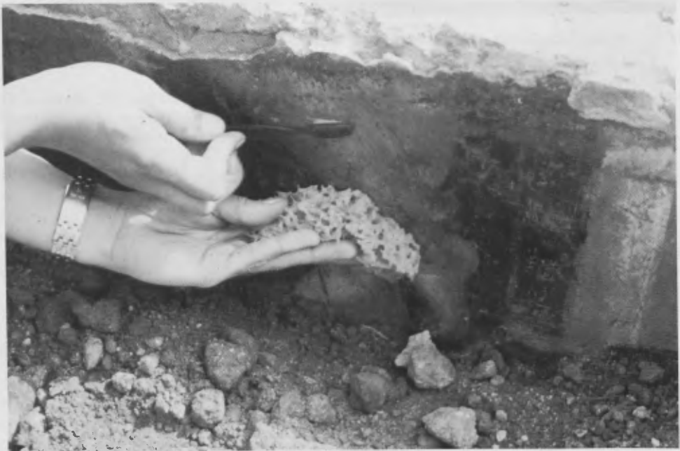
Figure 4. Cleaning: the intervention is restricted to removal of dirt residues from the painted surface. Photo: author.
