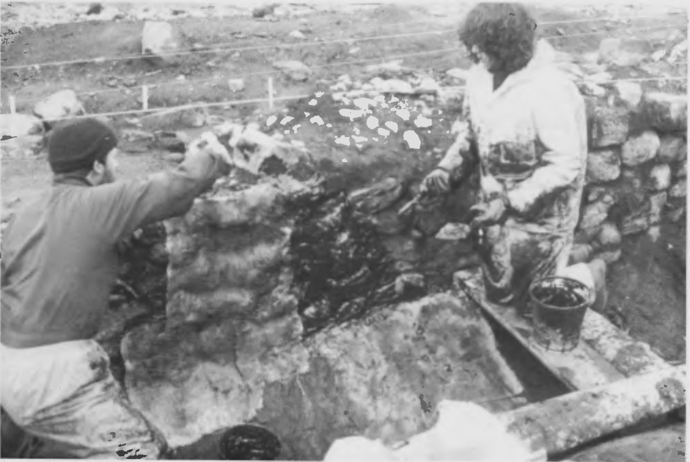
Figure 3. Applying polysulfide rubber to the wall.
