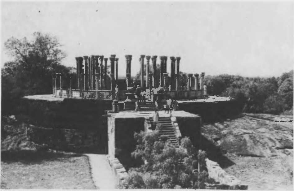
Figure 1. Vatadage at Medirigiriya after roof has decayed.
