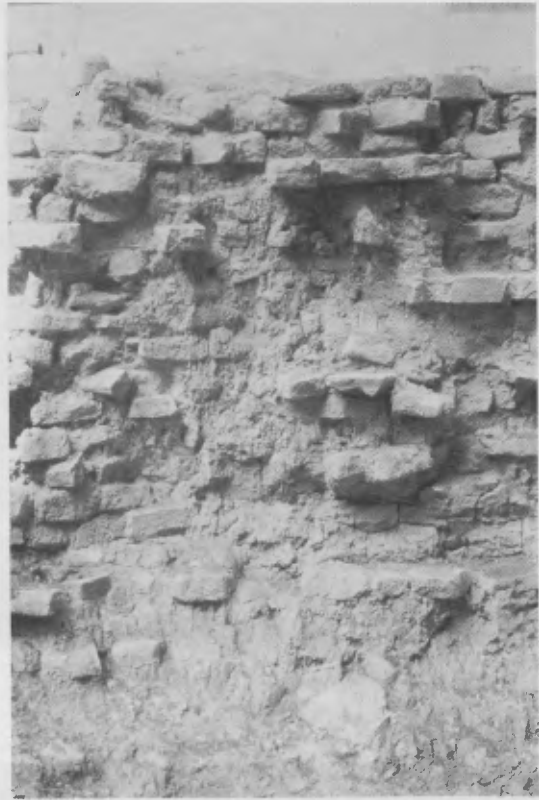
Figure 4. Detail of the wall excavated during the conservation intervention. The structure has maintained its original texture and consistency. Photo: author.
