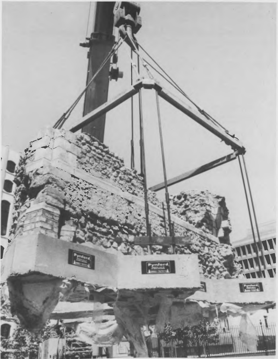
Figure 4. Mitre Street, City of London, 1984: a chapel from the church of Holy Trinity Priory, Aldgate, is lifted by special crane so that building works can commence on site; it was later lifted back into the same position, but slightly lower down. The chapel was underpinned with concrete and lifted in one piece (Museum of London).
