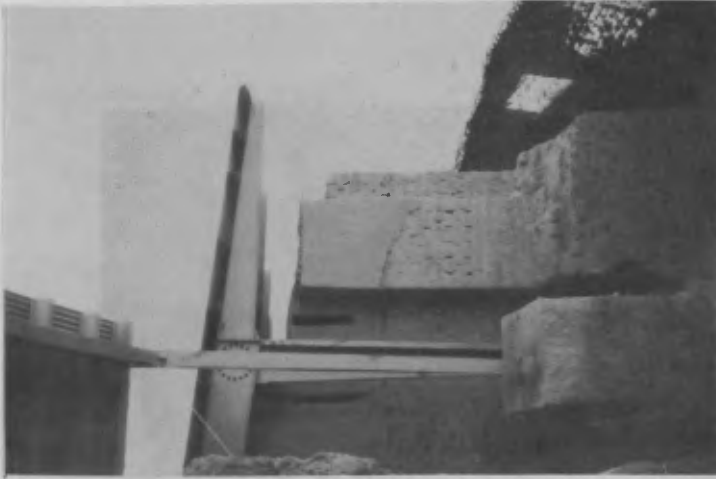
Illustrating a) steel roofs
