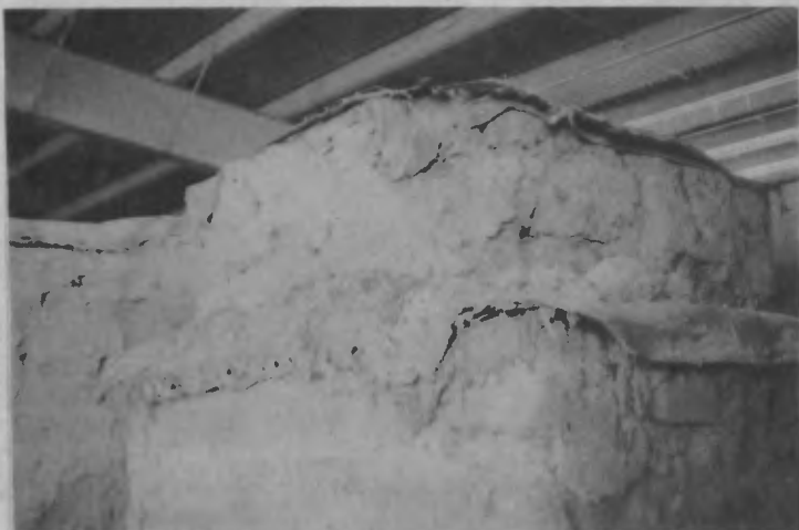
Capping using reed mats and kaghel with a layer of guni between.
