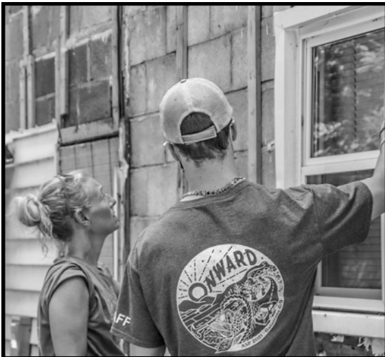
Courtesy of Appalachia Service Project -Home Repair
