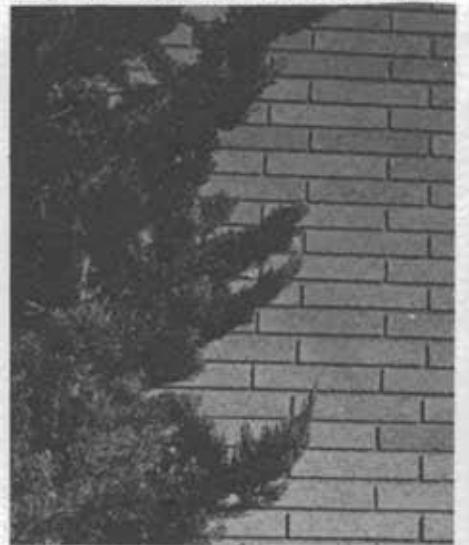
Norman face brick with ruffled texture in one-third bond using a raked joint.
