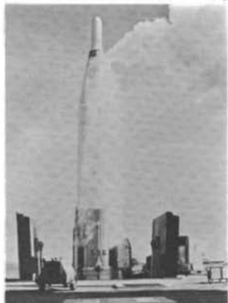
Atlas "F" missile in readiness, over silo built by Utah joint venture.
