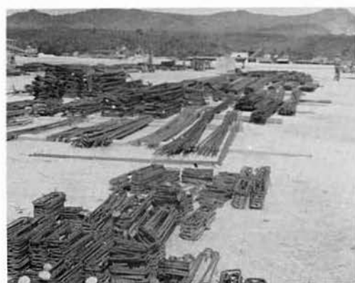
Stock-piled pre-fab re-bar.
