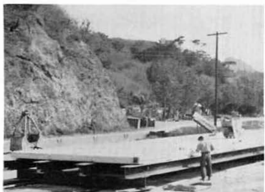
The precast Seaplane Ramp extension.
