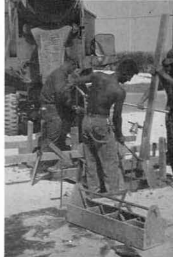
Get that concrete in the ground.
