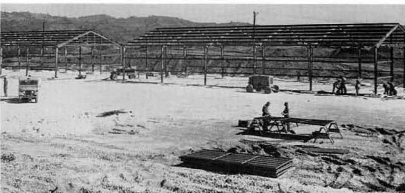
Two of the three steel skeletons await siding.
