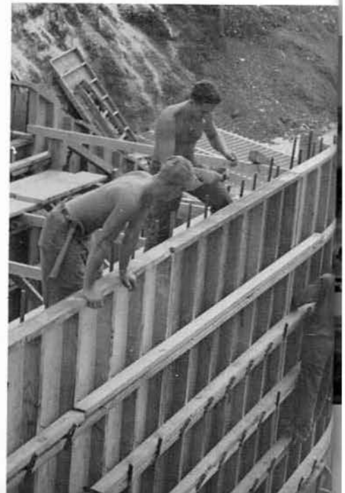
Working on the East Road Culvert.
