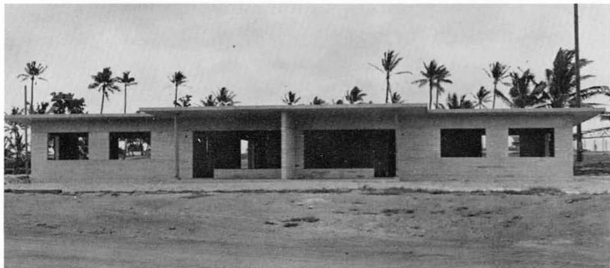
Completed except for interior work.
