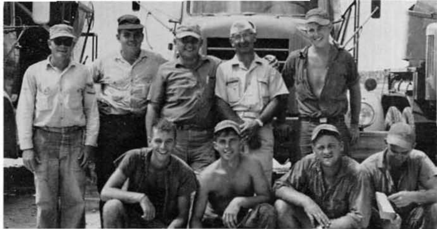
TM Crew. The men and trucks that hauled concrete from the Batch Plant to various parts of the island including many of the MCB ELEVEN projects.
