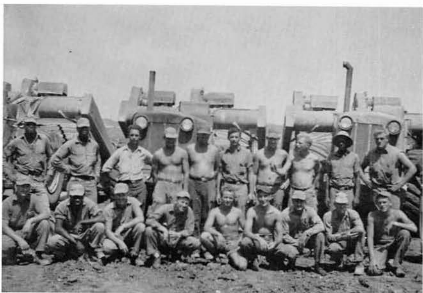
The men who handled the rough grade work.
