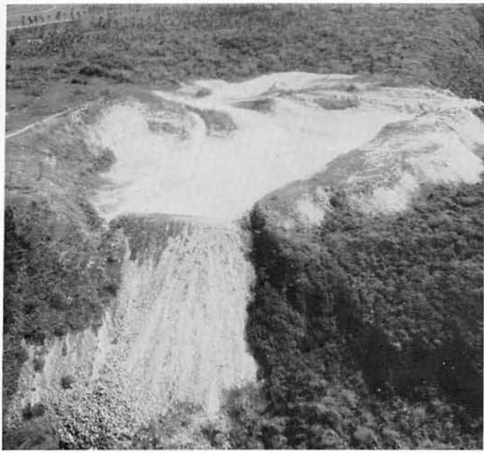
The Fadian Point Quarry where nearly 70,000 tons of coral were blasted loose and hauled to the crushers.
