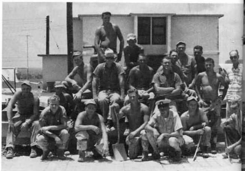
The Concrete Crew.
