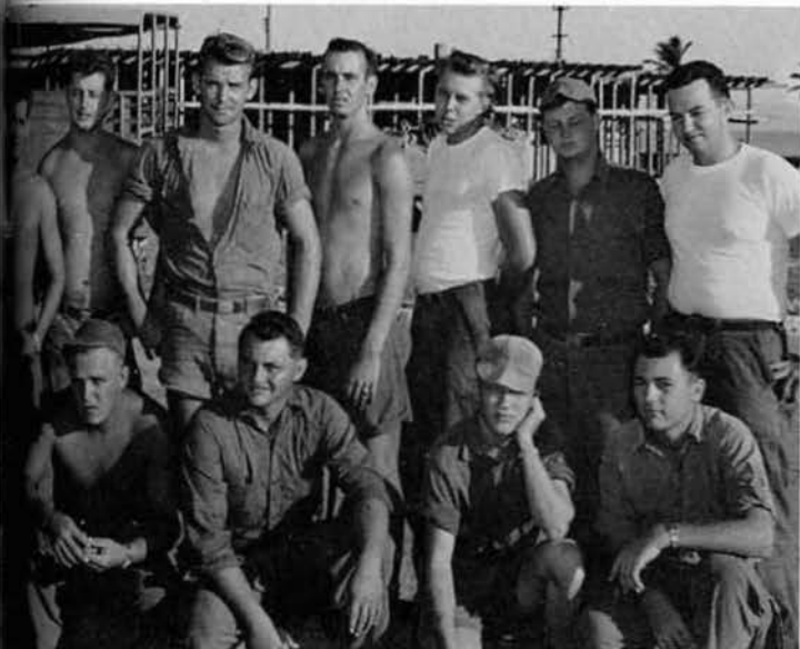
Pipe Plant Crew, who put out nearly three miles of pipe.
