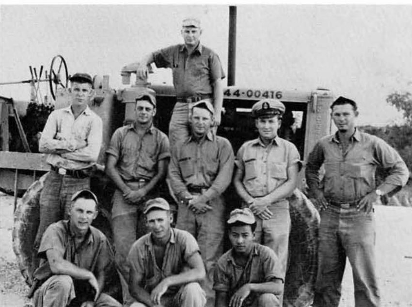
The Fine Grade Crew who put the finishing touches on the coral pads.
