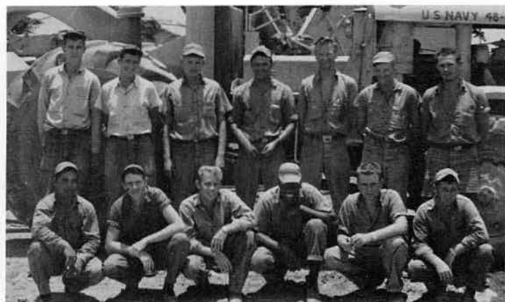
Part of the crew that hauled coral for pads. 95% compaction is like squeezing blood out of a rock, but they did it.
