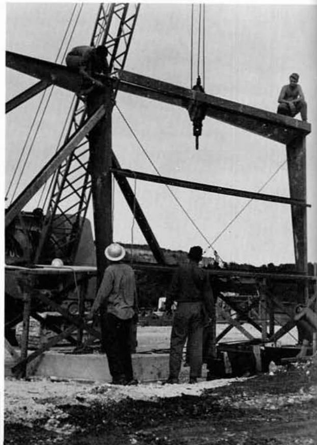
Soon the steel goes up.
