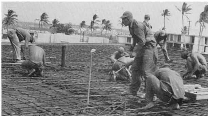
OK, let's get this cross-word puzzle finished and get some concrete up here.
