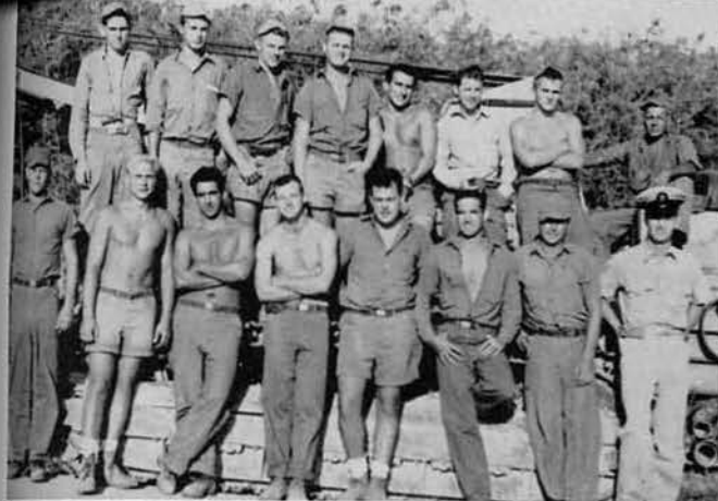
The Pipeline Crew.
