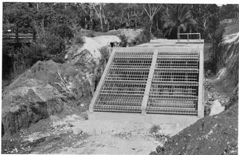
East Road Box Culvert.
