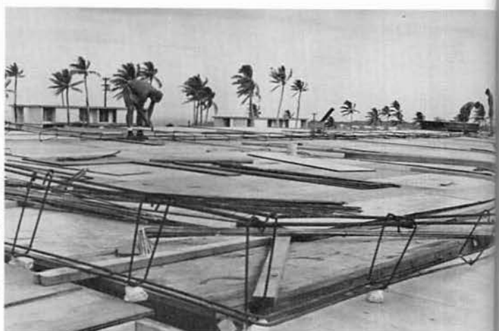
Preparing pre-fab re-bar for placement on the roof.
