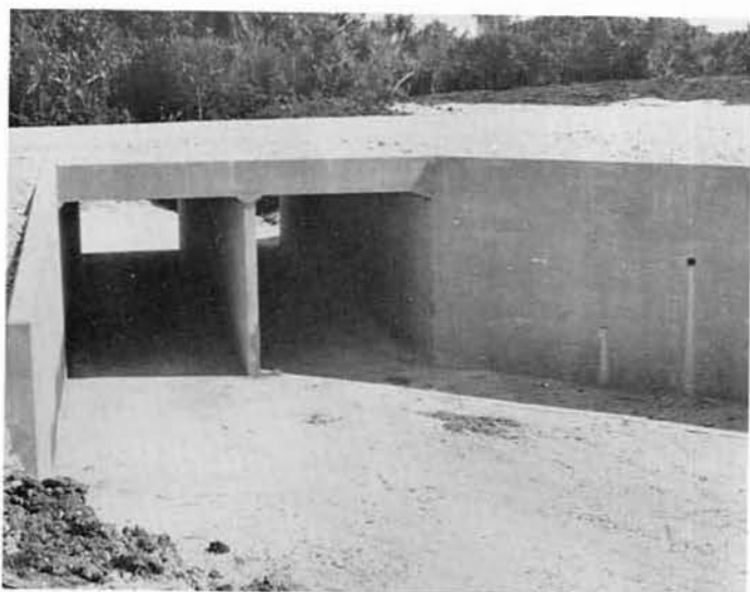
Norton Road Box Culvert.
