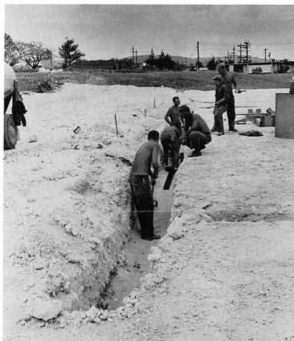
Dig out a ditch, lay some sewage line,
