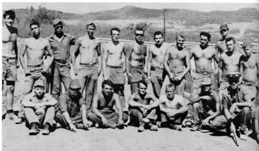
The Base Slabs Crew that put in the slabs for the Battery Charging Shop, Vehicle Storage Shed and the Paint Spray Building.
