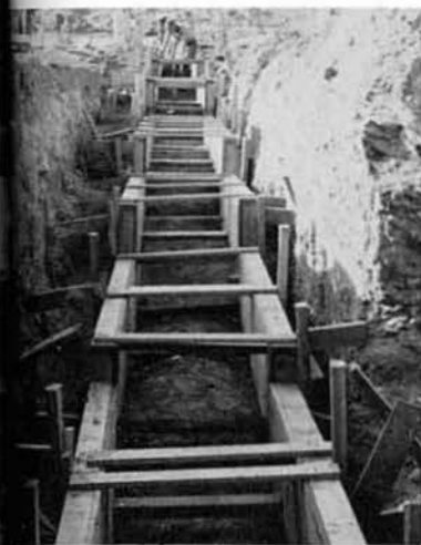
We got fancy with these footings.
