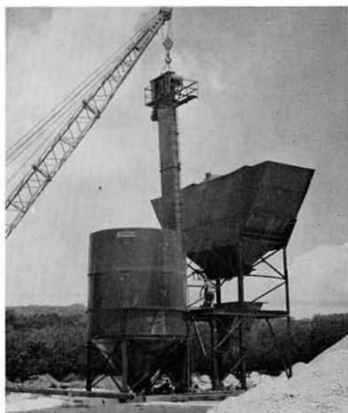
Final steps in the erection of the Batch Plant.
