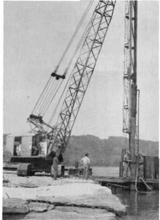
Not looking for oil, just driving a few piles.
