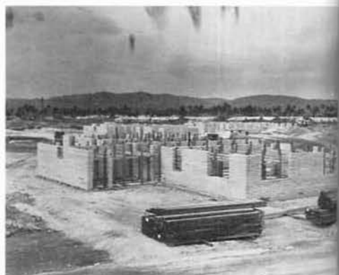
Up goes some bracing and staging.
