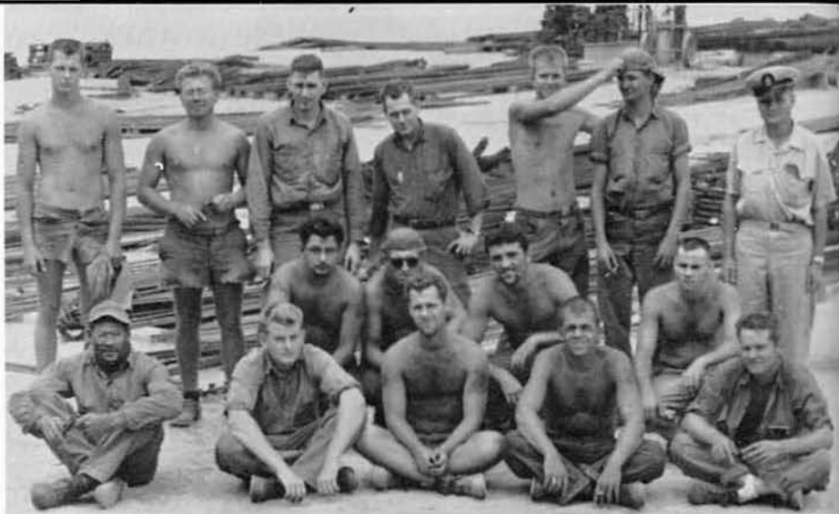
The pad's Steelworker crew.
