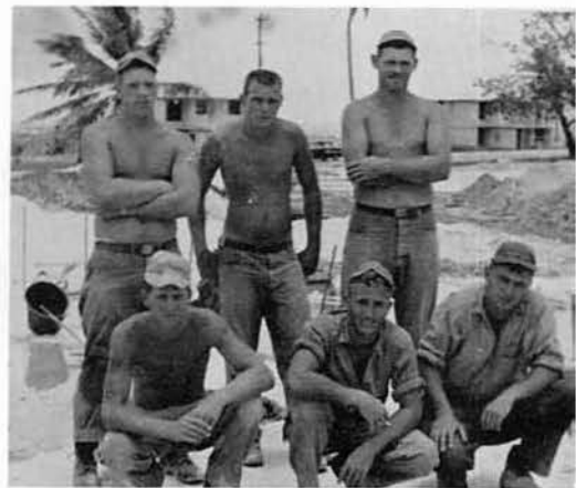
The Base Slab finishing crew.
