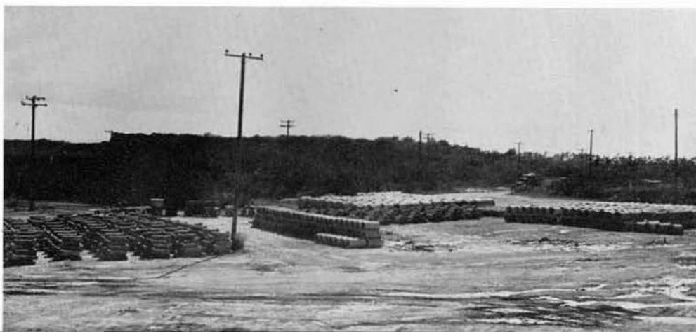
A small part of the concrete pipe produced.
