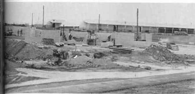
Things happened fast and block walls sprouted up overnight.
