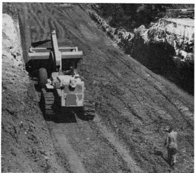
A bed for the Box Culvert.
