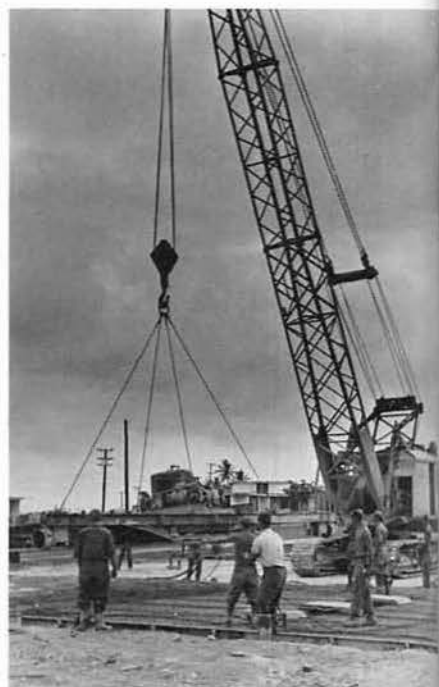
The base slab re-bar work is completed and the concrete crew moves in with their screeder.
