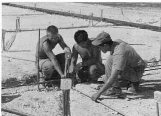
The coral pad is ready and conduit gets laid.
