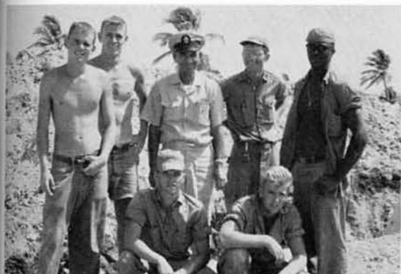
Sewage Line Crew. NAS's Sanitary Seven.
