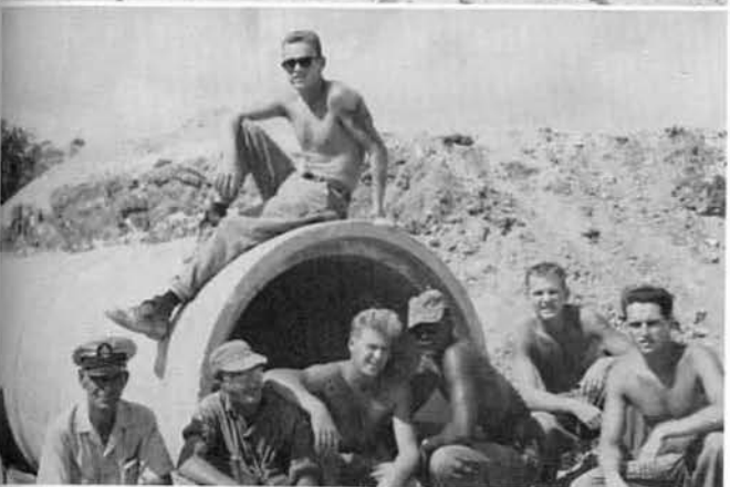
The Relief Culvert Crew.
