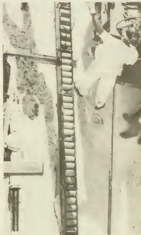
This is a section of a roller train, a series of rollers which keep rising stem valves in the locks culverts rolling, up or down, in spite of the heavy pressure of water against them.
