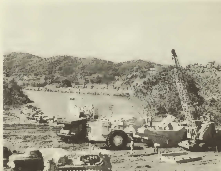
Mechanics begin final assembly of one of the big scrapers as unloading proceeds.
