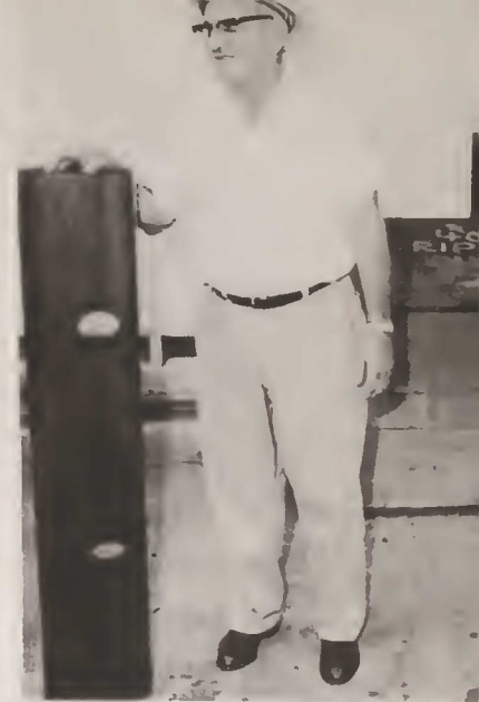
William Black, Maintenance Superintendent, Pacific Branch, with a section of the new rubber seal for bottoms of the lock gates. These heavy, tough rubber pieces weigh 19 pounds per foot. They're replacing thinner rubber strips fastened along the bottom edges of the gates.
