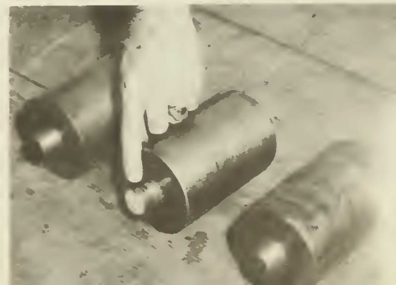
Three of the rollers which make up the trains. There are 61 rollers to each train, each train is 27 feet long and 2 are required for each rising stem valve. Finger points to worn trunnion, hand indicates relative size of roller.
