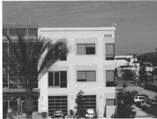
View toward TX antenna on rooftop from Site 1 at 10m AGL (zoom)
