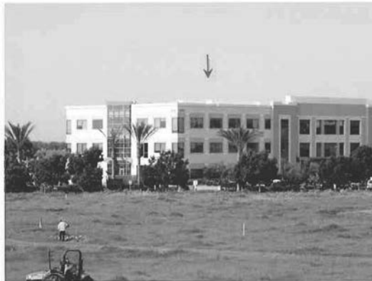
View toward TX antenna on rooftop from Site 7 at 10m AGL (zoom)
