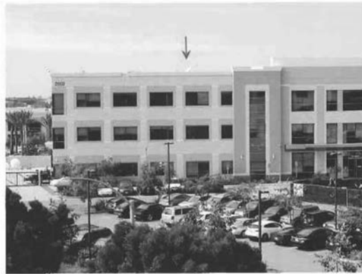
View toward TX antenna on rooftop from Site 3 at 10m AGL (zoom)
