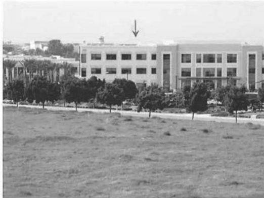
View toward TX antenna on rooftop from Site 5 at 10m AGL (zoom)
