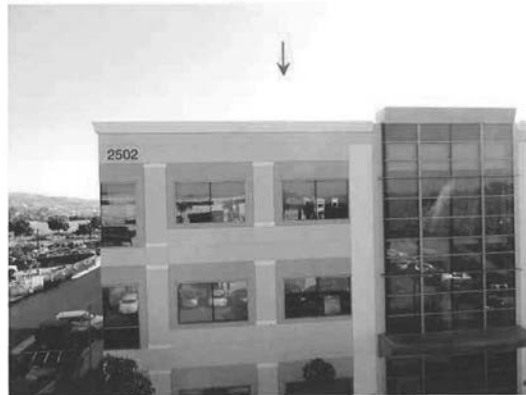
View toward TX antenna on rooftop from Site 11 at 10m AGL (zoom)
