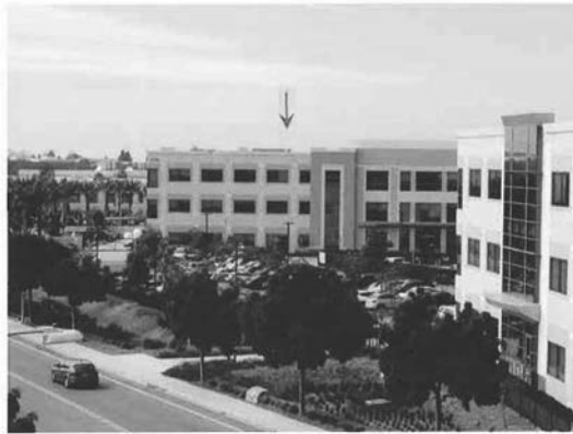
View toward TX antenna on rooftop from Site 4 at 10m AGL (zoom)
