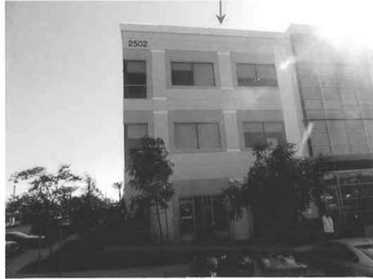
View toward TX antenna on rooftop from Site 11 at 2m AGL
