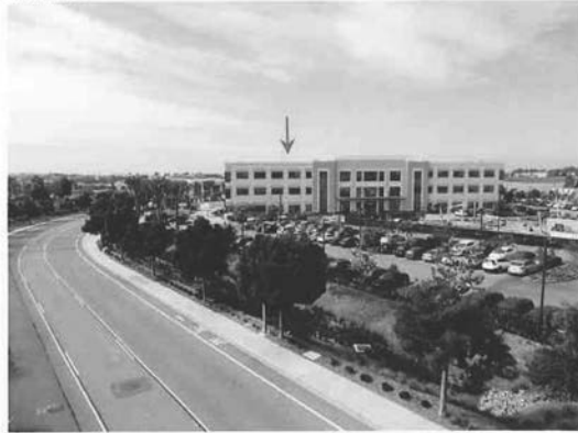
View toward TX antenna on rooftop from Site 3 at 10m AGL
