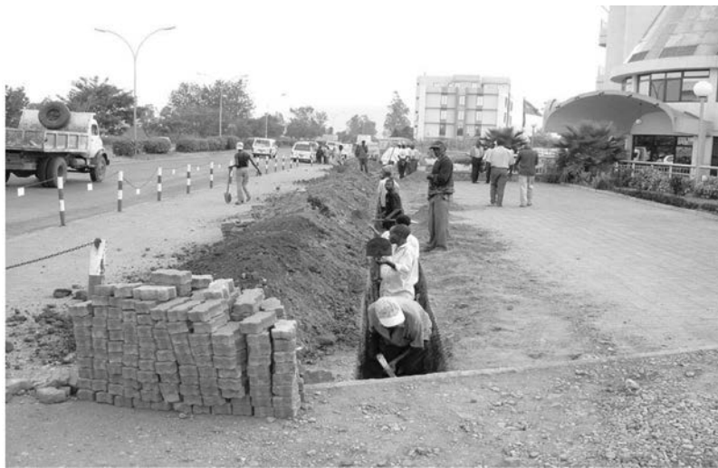
Figure 2: Fiber installation in 2003 in Kigali, Rwanda
