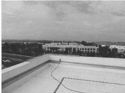
View from rooftop looking southwest
