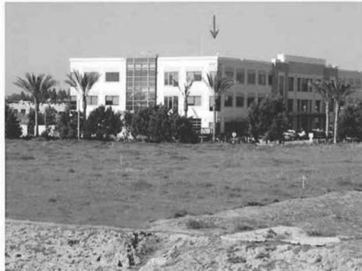
View toward TX antenna on rooftop from Site 8 at 10m AGL (zoom)
