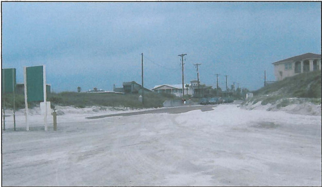
Vehicle Beach Access Point at Avenue G
