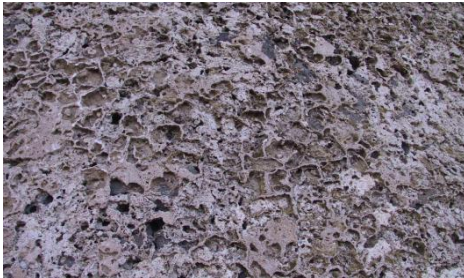
Fig. 14 – Torre di Foghe, tafones like- honeycomb in the exposed NO surface of the tower
