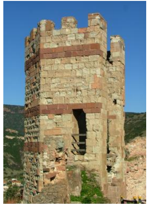
Fig. 4- View from SE of pentagonal tower.
