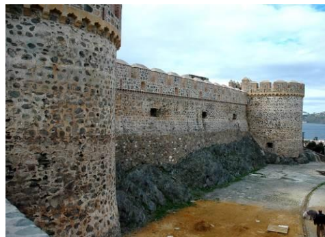
Fig. 6- Western stretch of the barrier of the Castle of Almuñécar. The original escarpment which no longer exists covered the rock that can now be observed.
