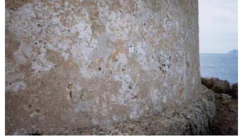
Fig. 3 - Northern side of the tower: wall covering partially restored
