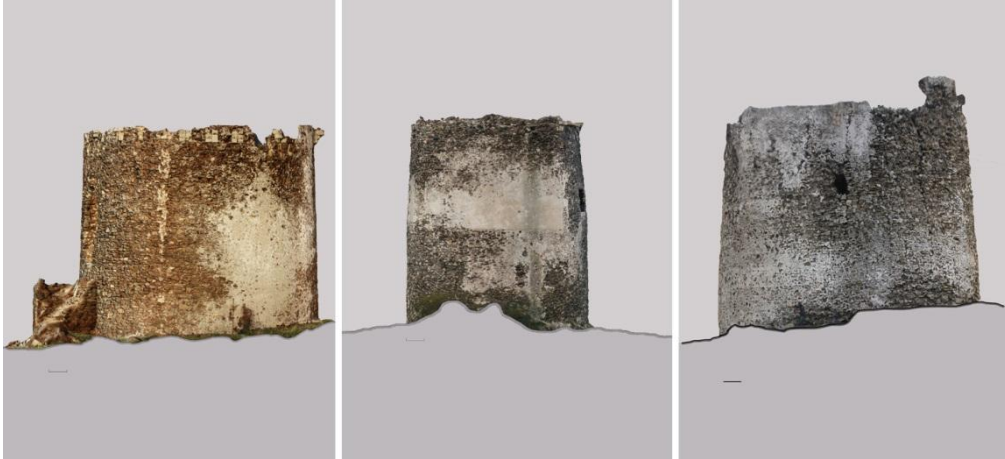
Fig. 1- Orthogonal perspective view of Trabuccato, Cala d'Oliva and Cala d'Arena towers obtained by processing the 3D model (Murru, 2015).
