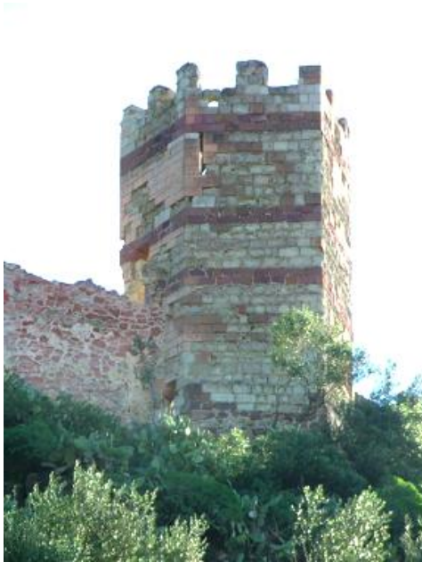
Fig. 3- View from NW of pentagonal tower.
