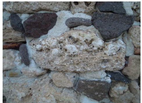
Fig. 11- Restoration Portland cement
