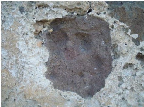
Fig. 8- Andesitic stones into bedding mortars
