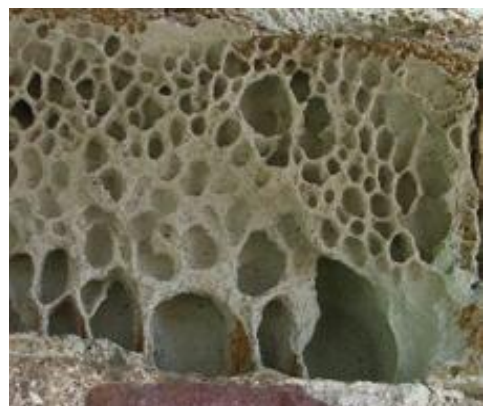
Fig. 6- Alveolation with different size of alveoli (15-80 mm) with lightly iso-orientation, related to different welding inside the same ashlar.
