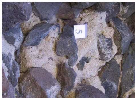
Fig. 18 - FOG-M5 sample – Bedding mortar
