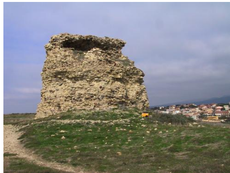
Fig. 2- Torre del Pozzo before the restoration
