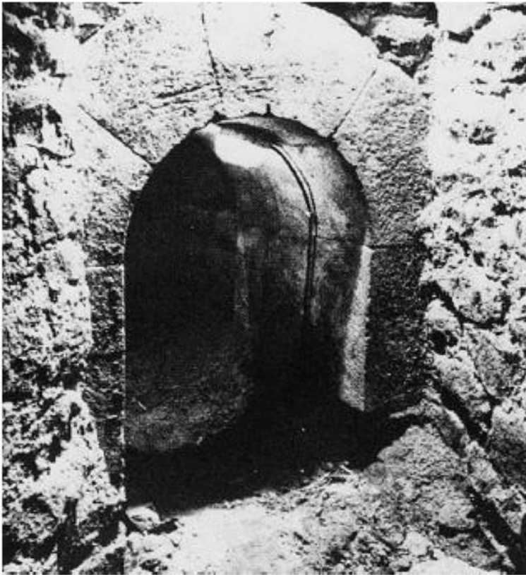
Fig. 1.6 Wastewater canal of a castle in Frankfurt from the 12th century, with direct discharge into the river Main (Grewe 1991).
