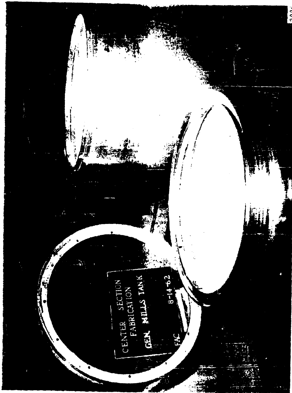
Figure 6.3 Bayonet Rings on Center and Tail Sections
