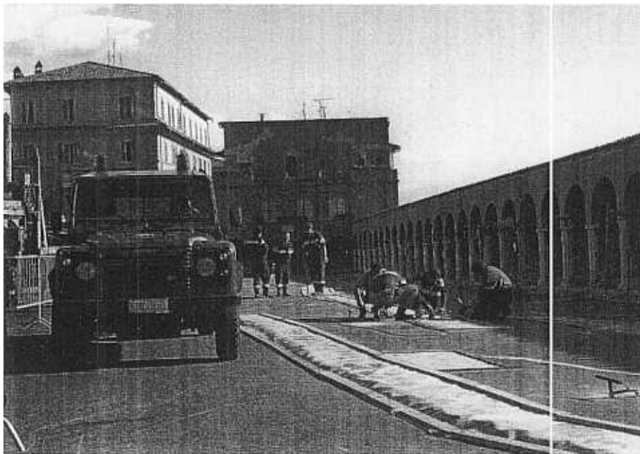
Figure 4 - In Assisi, significant cracks had opened in the Piazza Inferiore di S. Francesco, indicating earthquake-caused subsidence. The cracks had been covered with plastic (foreground). In this photo, soldiers are beginning to string cables to stabilize the arcade to the right in the photo.
