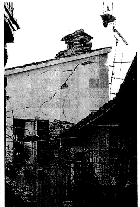
Figure 3 - This building in Nocera Umbra illustrates typical damage to stone buildings in the region.
