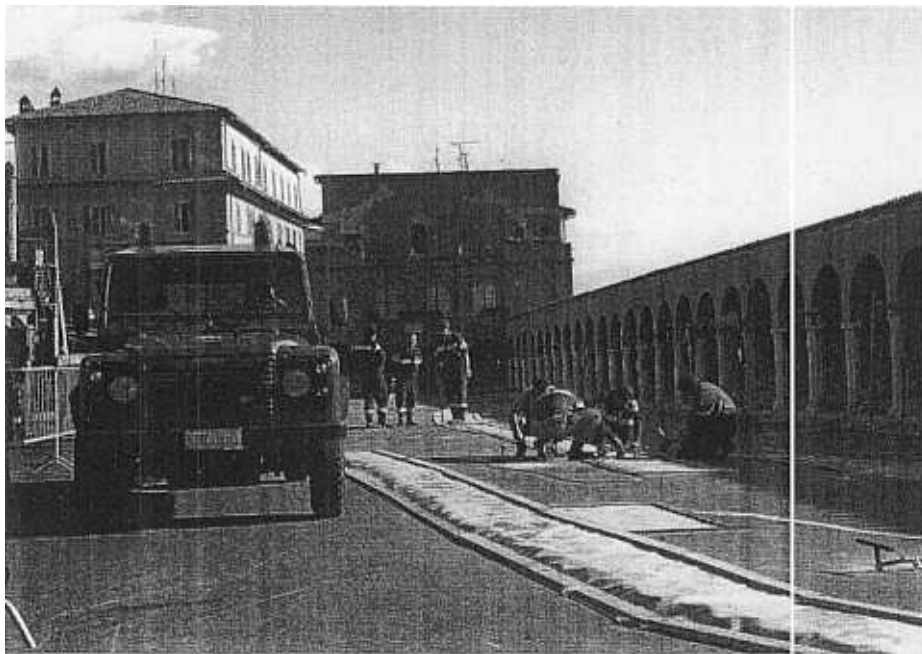
Figure 4 - In Assisi, significant cracks had opened in the Piazza Inferiore di S. Francesco, indicating earthquake-caused subsidence. The cracks had been covered with plastic (foreground). In this photo, soldiers are beginning to string cables to stabilize the arcade to the right in the photo.
