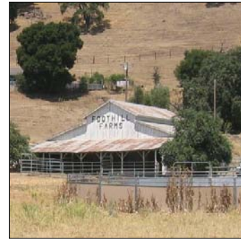
The barn at the base of Sunol Ridge serves as an acknowledgement of ranching activities during the American Farm Period.
