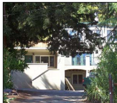
The Park includes a number of residences that are used as security residences and as a staff office/maintenance facility.
