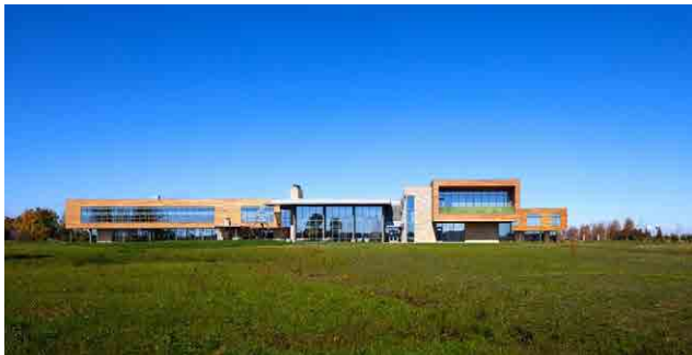
a) Exterior view of the building (view from South)
