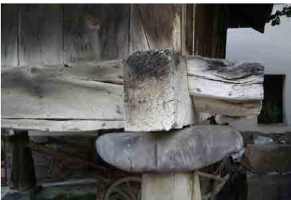
Figure 8. orreo corner detail. Asturias and Galicia, Spain. Source: (iberianature.com N. Lloyd)
