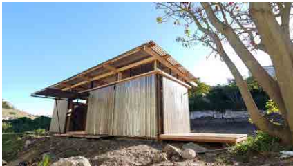
Figure 1. The Community Makerspace in Port Elizabeth, South Africa was constructed almost entirely of reclaimed materials, at a cost of $1500 in under 7 days by a team of 11 (Shall 2019).
