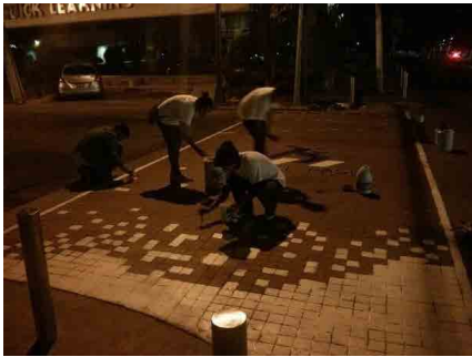
Figure 3. Painting crosswalk. Source: (Esteller 2015)
