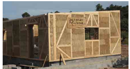
Figure 1. Construction process using rice straw panels.
