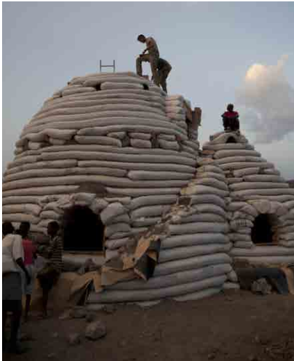
Figure 5. Figure 5: Superadobe sandbag shelters in Djibouti in 2012
