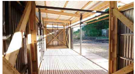
Figure 1. The Community Makerspace in Port Elizabeth, South Africa was constructed almost entirely of reclaimed materials, at a cost of $1500 in under 7 days by a team of 11 (Shall 2019).
