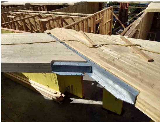
Figure 8,9. The Canyons CLT and light frame integration. Source: (Marcus Kauffman, Oregon Dept. of Forestry n.d.)
