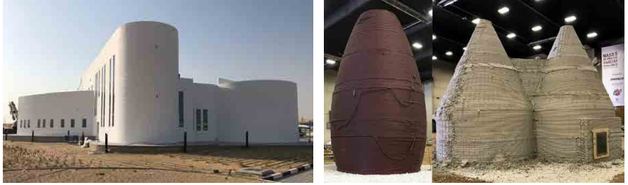
Figure 4. Examples of 3D-printed construction; office building in Dubai (left); constructions in NASA contest (right). Sources: ( https://www.apis-cor.com/ , https://spectrum.ieee.org/tech-talk/aerospace/space-flight/3d-printers-could-build-future-homes-on-mars , photographer Tracy Staedter)
