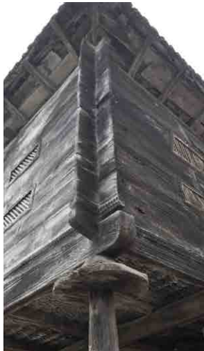
Figure 9. Post/ head/ disk/ and loggia detail. Source: (Author 2014)
