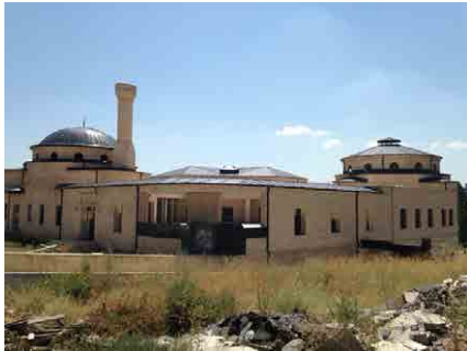
Figure 1. The abandoned condition of the mosque- cemevi complex
