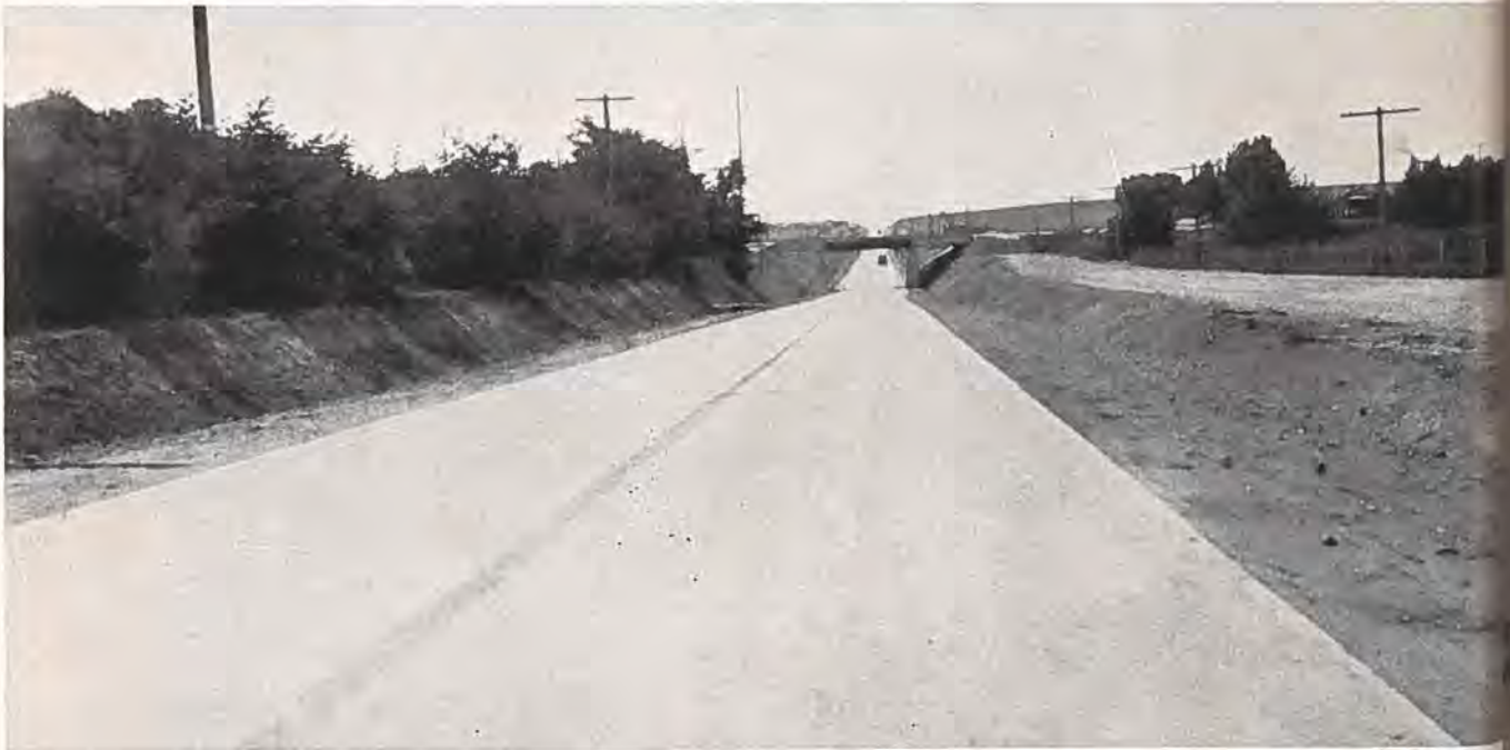
A long stretch of the Federal Aid concrete pavement east of Boulder, showing newly completed underpass of the C. & S. railroad tracks at the foot of Goodhue hill. Photo by U. S. Bureau of Public Roads.
