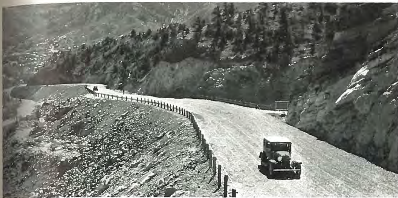
Picture above shows a section of the magnificent new highway through Ute Pass, above Manitou in El Paso County, constructed by the Colorado Highway Department in co-operation with the U. S. Bureau of Public Roads. Elimination of sharp curves and steep grades, with gravel surface, now make driving a pleasure. Photo by H. L. Standley, Colorado Springs.
