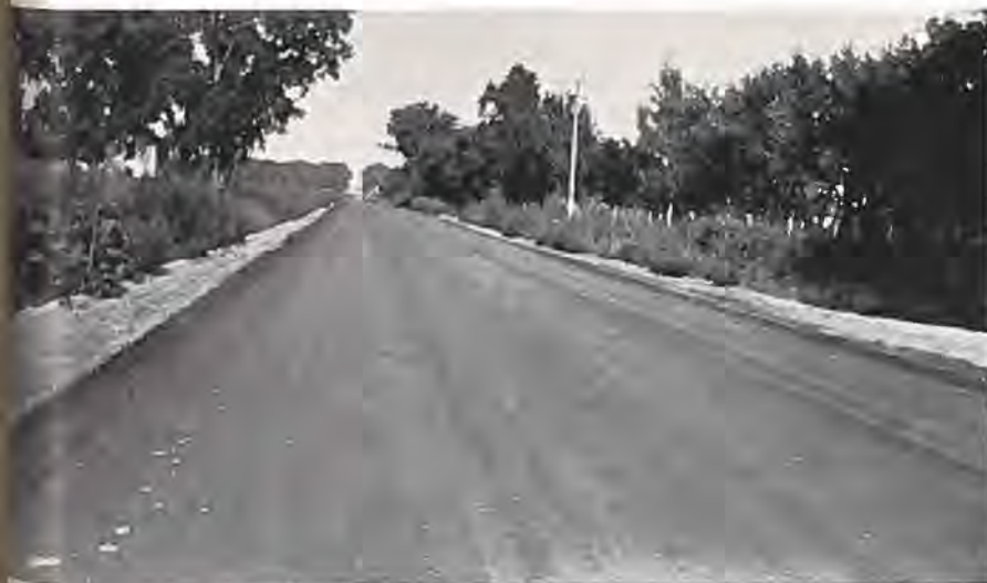
The "finished product," showing road northwest of Fort Collins after it had been "given" to traffic two weeks. Photos by Paul J. Greer.
