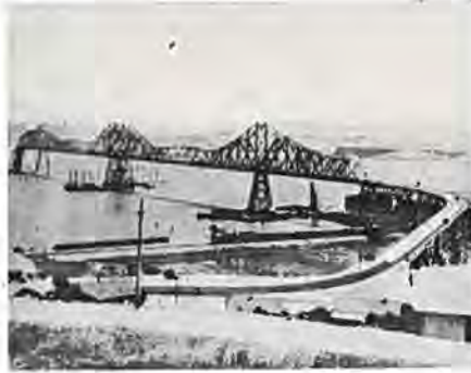
Carquinez Strait Bridge—Spanning Carquinez Strait, California. Two 1,100-ft. cantilever spans. Deep-water foundations. Silicon steel compression members and heat-treated eye-bars. Proportioned for earthquake forces and designed with special protective details. Completed 1927.
