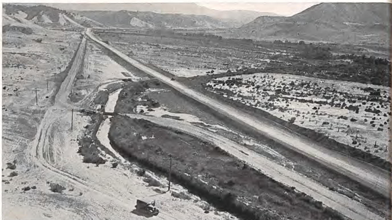
A section of the newly completed Federal Aid highway located east of Montrose, Leading to Cerro hill. Photo by U. S. Bureau of Roads.
