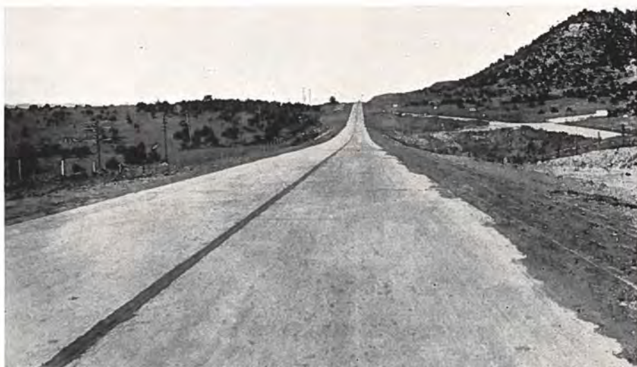
A section of the newly completed concrete paved roadway leading south from Trinidad in Las Animas County. Photo by U. S. Bureau of Roads.
