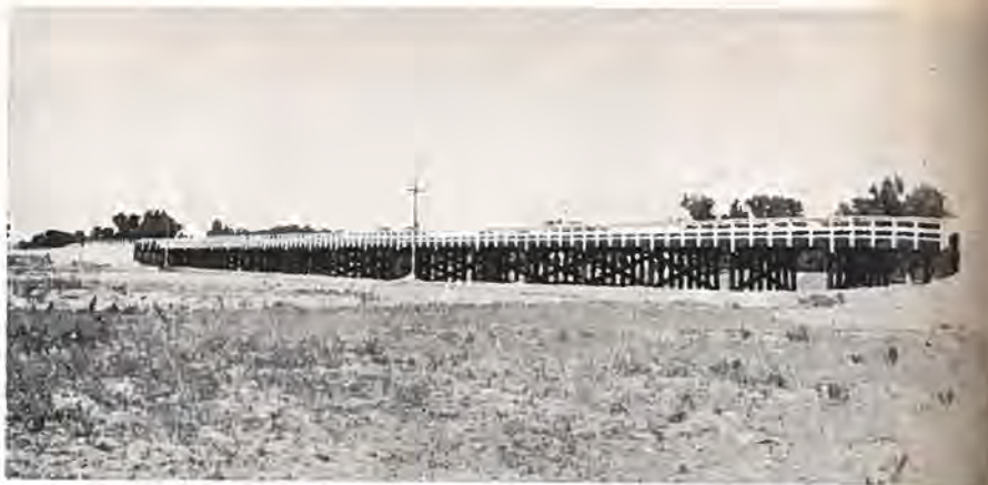
One of the splendid new creosoted wooden trestle bridges located on the Denver-Limon highway, over 200 feet in length.
