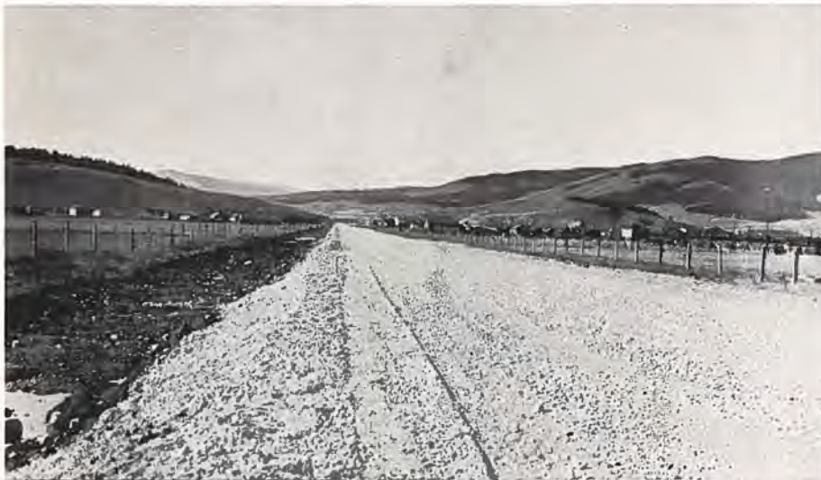
Showing a stretch of the new graveled highway between Fraser and Tabernash on the Victory Highway, completed during the 1931 construction season. Photo by U. S. Bureau of Public Roads.
