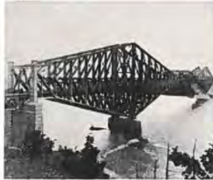
Quebec Bridge, crossing the St. Lawrence River. The world's longest cantilever span. Span 1,800 feet. Completed 1917.
