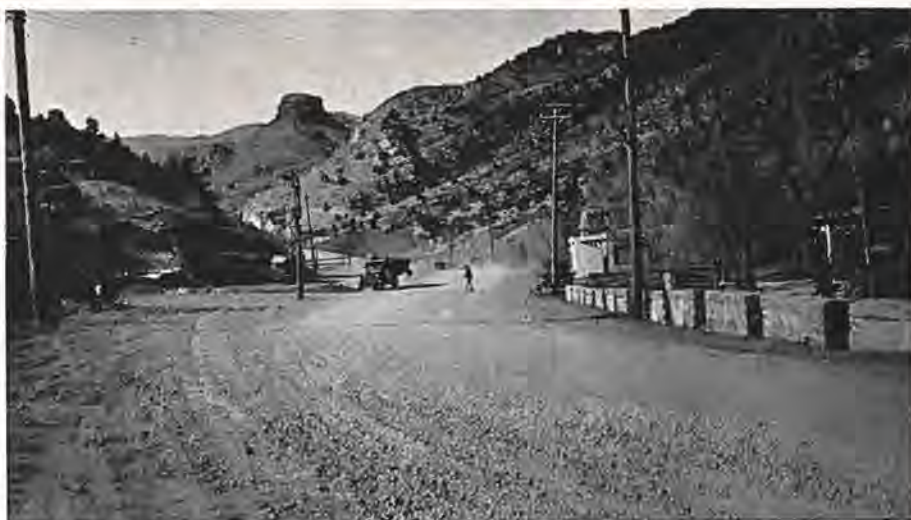
Showing entrance to new highway on left, old road on right, at Manitou end of project. Photo by V. H. Littlefield.
