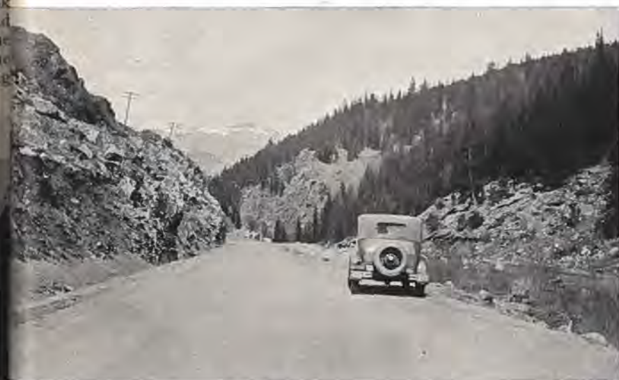
Section of the newly completed standard Federal Aid highway on Kenosha Pass in Boulder County, constructed by the State Highway Department, eliminating the steepest grade between Denver and the western slope. The old grade over this two-mile section was almost prohibitive in low for most cars.
