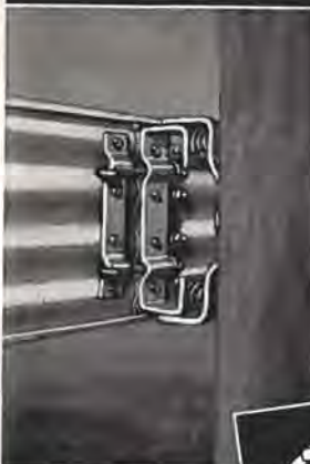
Above: Complete panel joint.
