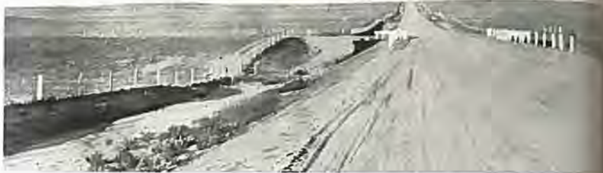
Above picture shows a stretch of the new highway extending east of Sterling, completed in 1931 with state and Federal Aid funds. The project was sixteen miles length and was constructed for oil surfacing. Photo by U. S. Bureau of Public Roads.
