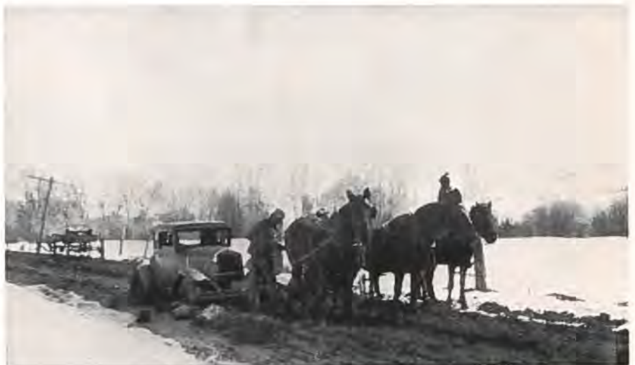
This is what the old road pictured on page 6 looked like in wet weather. Yes, these days are gone forever. Photo by U. S. Bureau of Roads.
