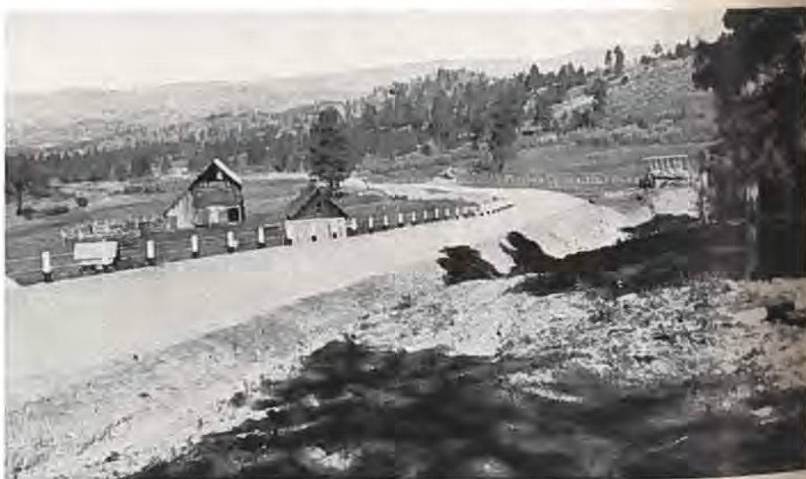
Showing a section of the new Federal Aid highway over Yellow Jacket hill recently opened to traffic. This can be traveled in any sort of weather. Photo by U. S. Bureau of Roads.
