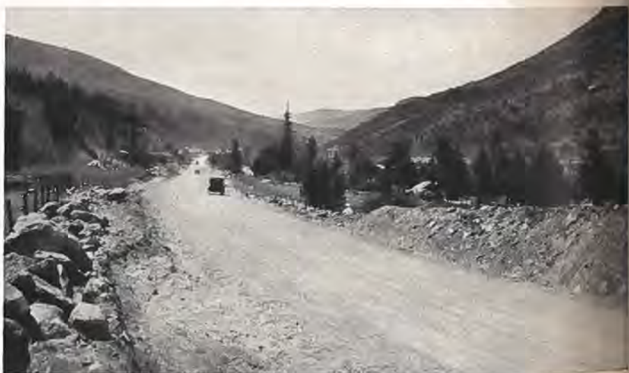
An example of gravel-surfaced highway located near Avon in Eagle County, constructed under Federal Aid specifications. Photo by H. L. Jenness.
