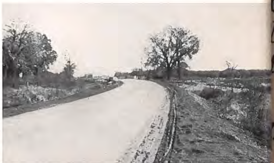
View of the new concrete paved Federal Aid highway located west of Fowler on the Santa Fe trail. Photo by U. S. Bureau of Roads.
