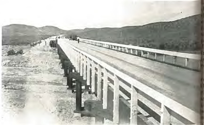
One of the scores of treated timber bridges constructed on the new Federal gravel surfaced highway extending thirty-five miles west of Craig on the Victor Highway. Photo by U. S. Bureau of Public Roads.
