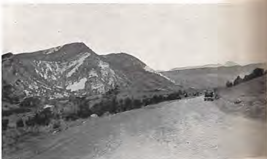
A section of newly-completed Federal Aid gravel-surfaced highway located east of Durango in La Plata County.
