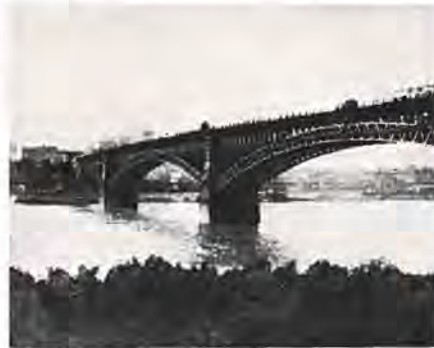
Eads Bridge—Steel arch bridge—over the Mississippi at St. Louis. Spans: 502, 520, 502 feet. Completed 1874.
