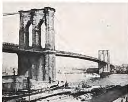
Brooklyn Bridge over the East River, New York. Span 1,595½ feet. Completed 1883.
