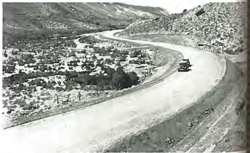
A stretch of modern Federal Aid highway located east of Montrose on U. S. road No. 50, which will save motorists thousands of dollars in "mud tax" in years to come.
