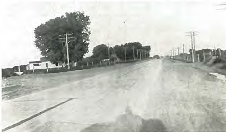
A beautiful piece of concrete pavement located west of Manzanola in Otero County on the Santa Fe Trail or U. S. route No. 50, constructed with Federal Aid funds. Photo by U. S. Bureau of Roads.
