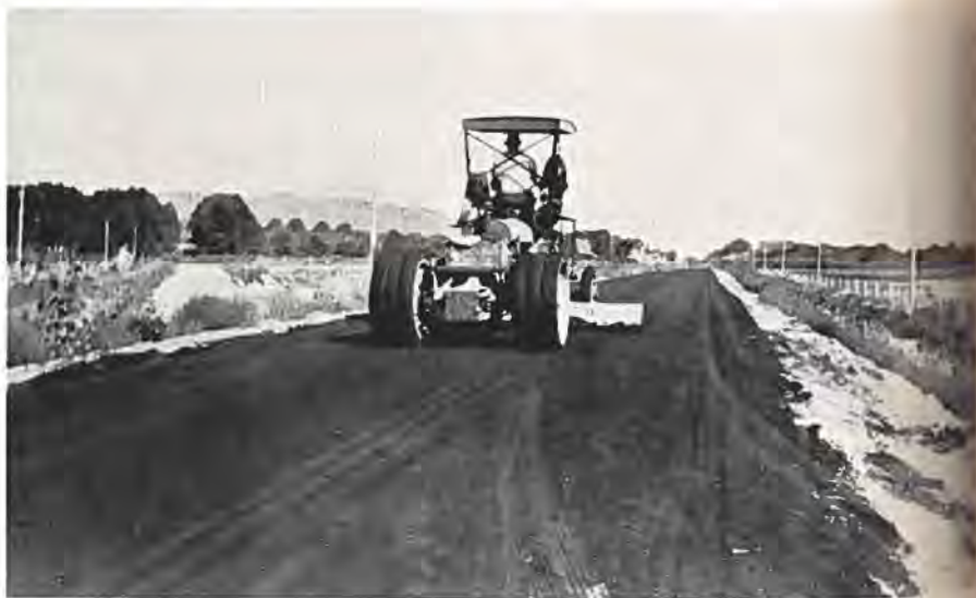
State motor grader smoothing oil-surfaced road northwest of Fort Collins, one of Colorado's low-cost surfaced highways.
