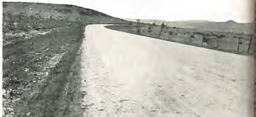
A stretch of oil-surfaced highway extending east from Trinidad in Las Animas County constructed by the State Highway Department under agreement with the U. S. Bureau of Public Roads.
