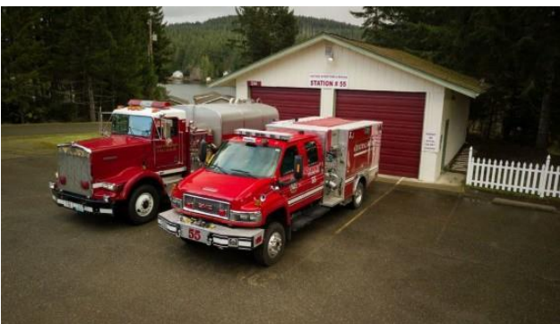
Lake Tahuyeh Community Fire Station – Built 1973
