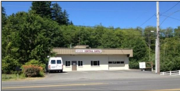
Central Supply – Built 1958
