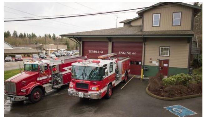
Chico Community Fire Station – Built 1999
