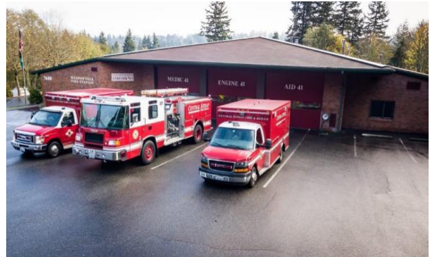
Meadowdale Community Fire Station – Built 1979
