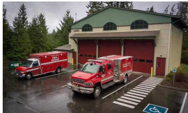
Island Lake Community Fire Station – Built 1999
