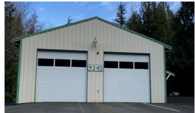
Facilities Maintenance Building – Built 1998
