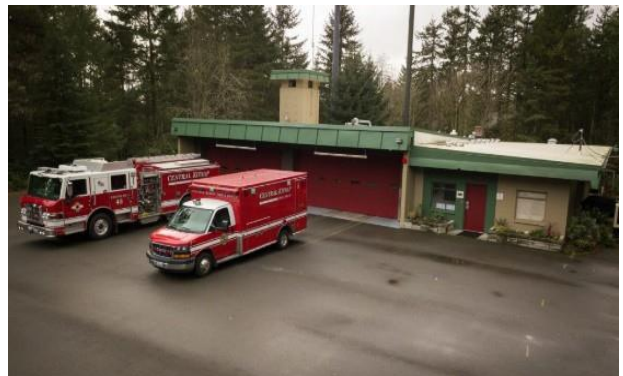
North Perry Community Fire Station – Built 1965
