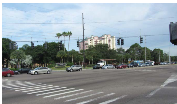
Northbound Queuing at Meadow Creek Drive
