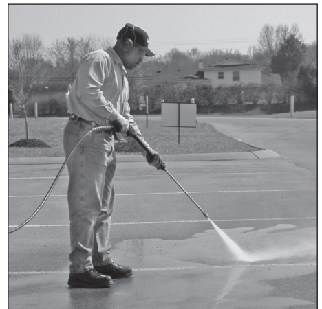
Figure 19 - Optimum angle to cleaning surface
