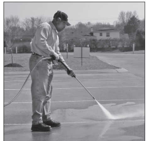
Figure 19 - Optimum angle to cleaning surface
