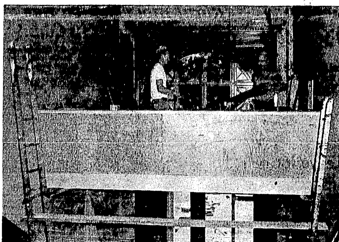
TO PROVIDE SPACE for the county clerk's office a mezzanine is being constructed above the front entrance to the court house at Mason. The exterior appearance of the building will not be changed, but inside a mezzanine will overhang the stairway leading to the main floor. A door will be cut through the wall on the north side of the mezzanine office can be entered directly from the clerk's office. The additional space will be used for the new Burroughs bookkeeping machine recently installed. At a meeting in Mason last week the board of supervisors authorized construction of the mezzanine office. In this picture Charles Knipfer (left) and Clifford A. Watkins, carpenters employed by Capital Roofing Co., Lansing, are shown at panning work. (News photo.)
