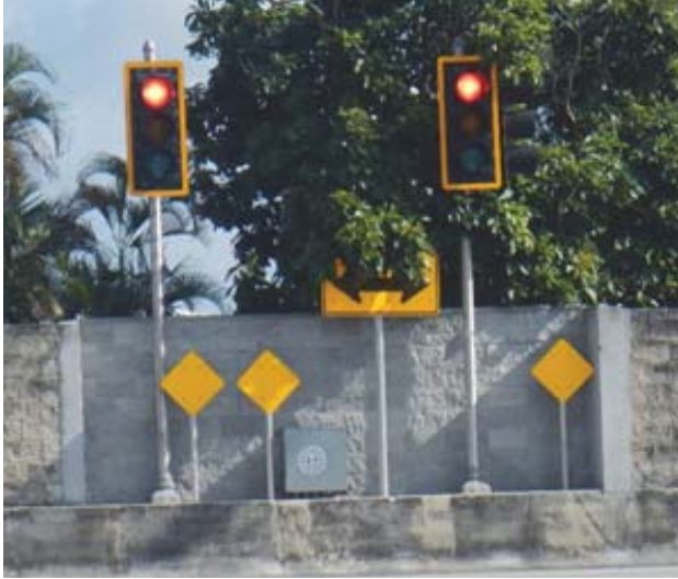
Copans Rd. and NW 3rd Ave. Signal infrastructure within a barrier wall own by the County. The wall also indicated the limits of the ROW.
