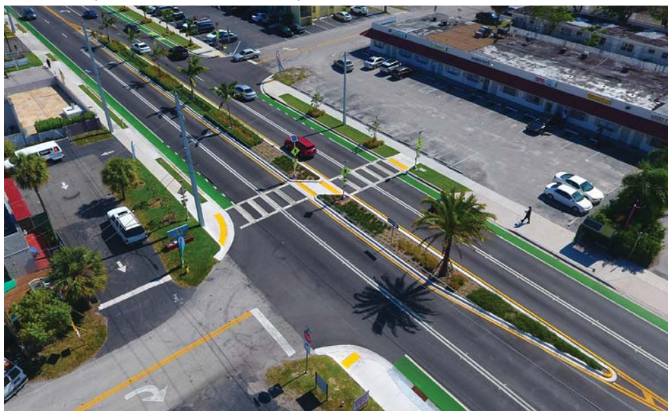
Andrews Ave. MidBlock Crosswalk
