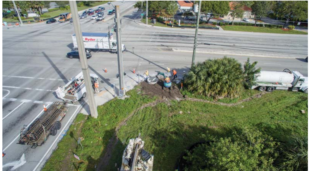
Commercial Boulevard and Nob Hill Road
