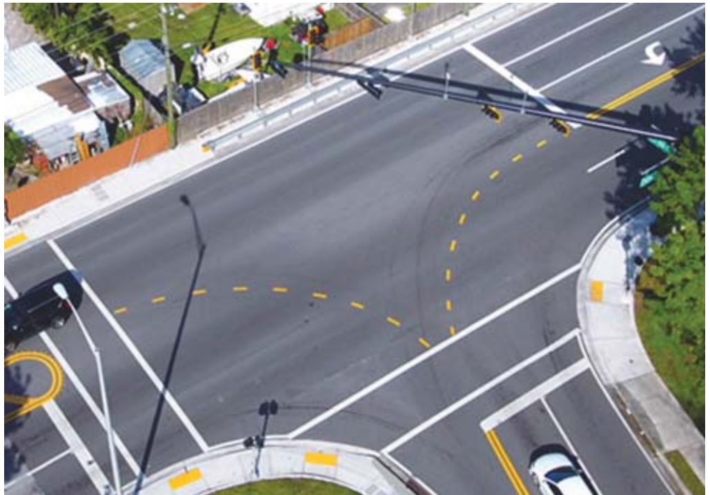
Peter Rd. and SW 46 Ave., T intersection, One diagonal arm along with ground mounted signal heads helped accommodate ROW issues.
