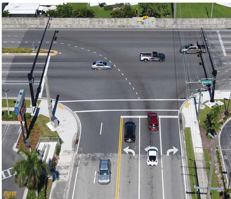
Copans Rd and NW 3rd Ave
