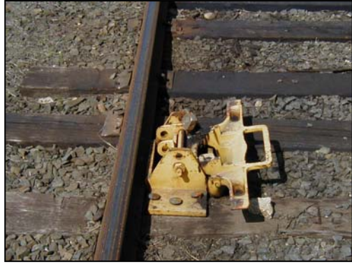
(23) Hinged Block Derail
