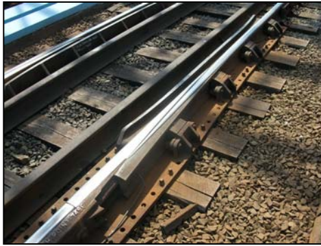
Sliding Rail Expansion Joint
