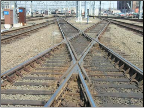
(17) Bolted Rail Crossing 2 - Rail Design
