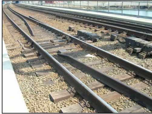
(22) Single Point Switch Point Derail
