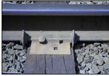
Conventional Tie/Creeper (Box Anchor)
