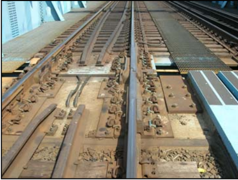
Two-Piece Manganese Steel Miter Rail
