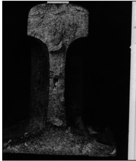
Defective Electric Flashbutt Weld from Iron Oxide Entrapment
