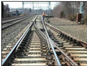
Rail Anchoring of Turnouts
