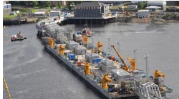
Clyde naval base - Astute Class jetty
