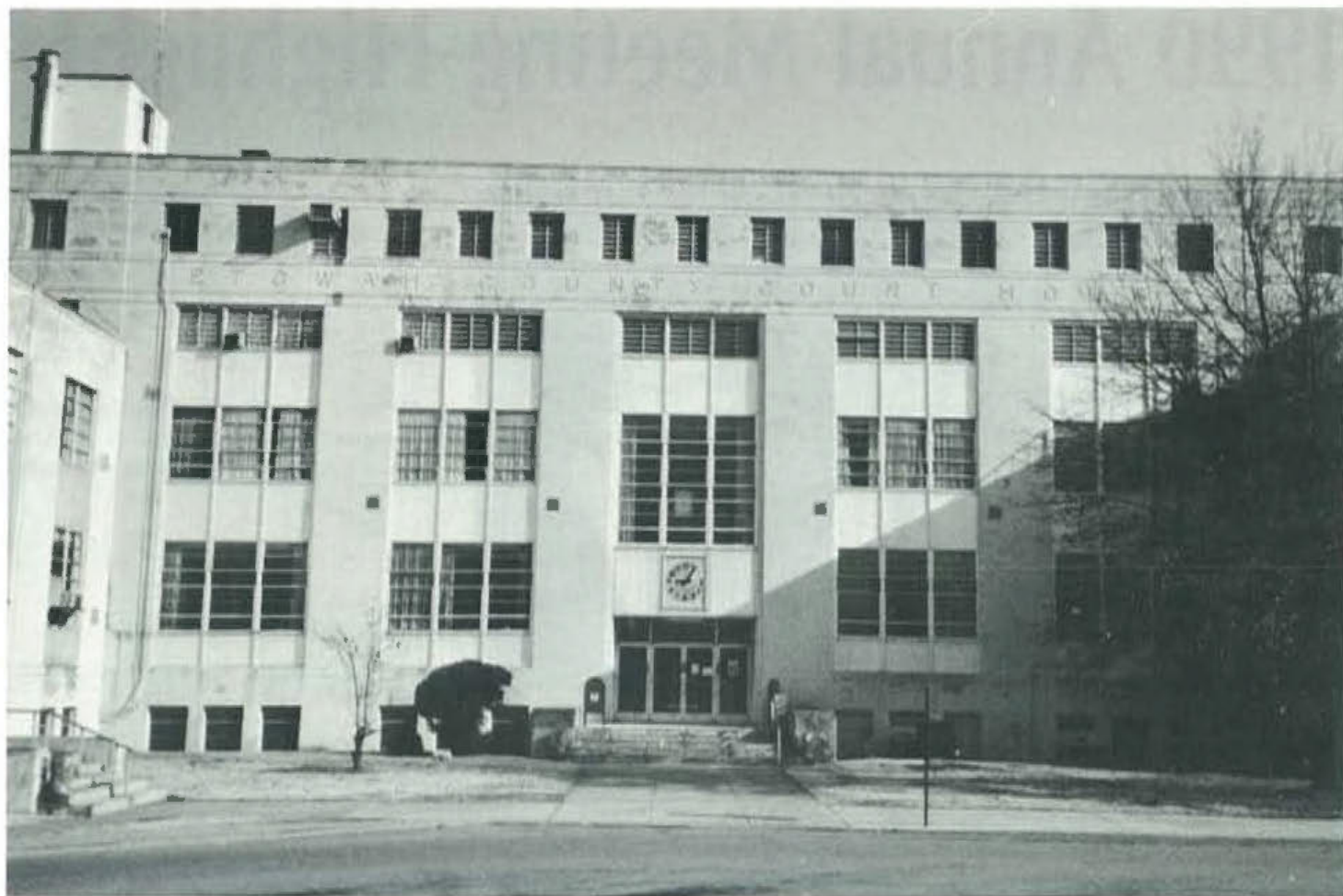
Etowah County Courthouse
