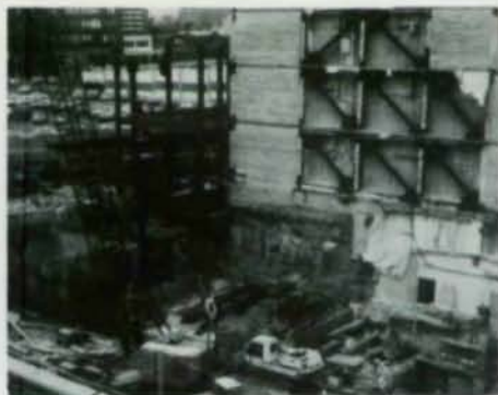
Fig. 4. Foundation work begins for new tower—with minimal disturbance to patients.
