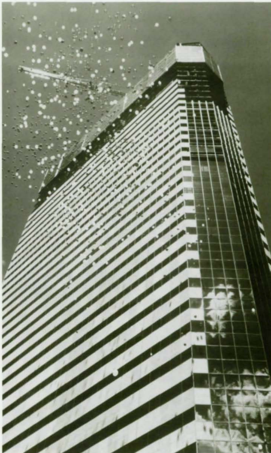
1999 balloons were released to celebrate topping out of 1999 Broadway Building, Denver, Colo. The 43-story office tower, built around a church, faces business district and famed Pike’s Peak.
