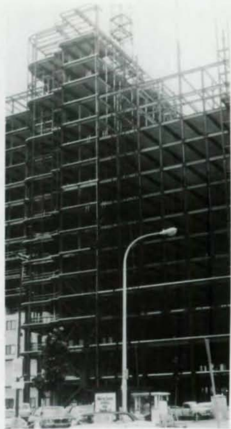
Fig. 7. Steel frame of new tower nears completion.
