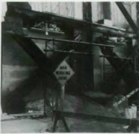
Fig. 6. Detail of wind bracing
