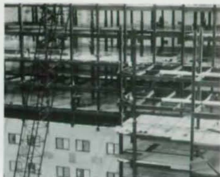
Fig. 5. High-strength steel framing extends over existing structure.
