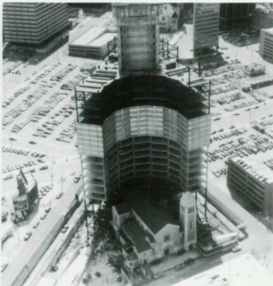
Rendering (l.) shows relationship between tower and church. Structural steel frame at mid-point (above). Three levels are enclosed by environmental screen. Self-climbing jump-form system, here 8 stories above steel, formed core.
