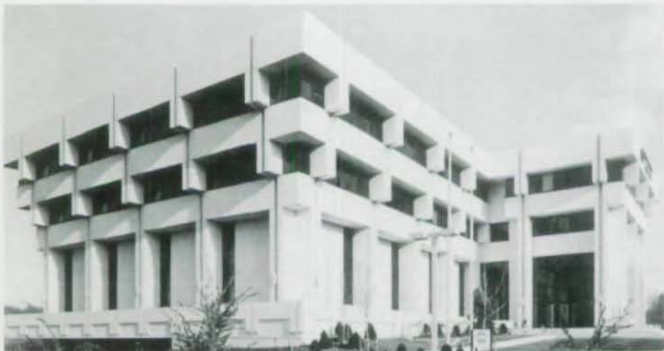
Energy-efficient Citizens First Bank, Glen Rock, N.J. headquarters. Shading and sun control accomplished with steel-framed cantilevers at 3rd and 4th levels. Designed by Tellefsen & Mader Associates.
