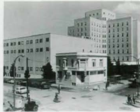
Fig. 2. Site prior to construction. Building in front was demolished; 5-story existing structure on left.
