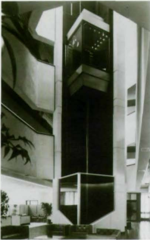
Dramatic atrium (l.) of Woonsocket Savings, designed with steel frame, has size reduced at each floor to increase usable space. Park Place, (r.), Clayton, Mo., built by Paric Corp., features steel-framed balconies overlooking park.
