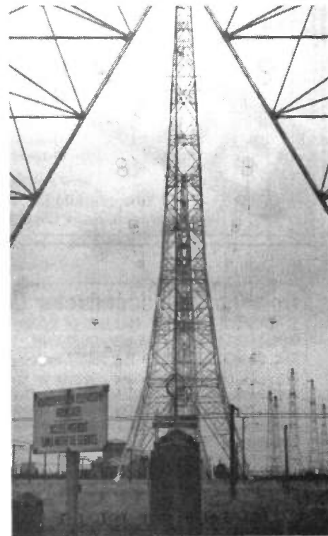
Antenna towers at Radio France International's transmitter site at Issoudun
