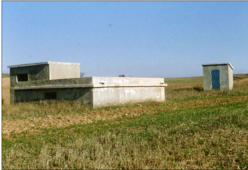
Well where the water comes out for the whole town. 1977. Photo provided by Federico Varona
