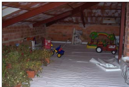
Attic of a modern house. 02/10/2006
