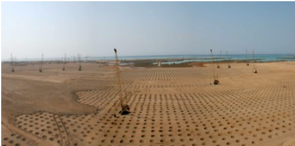
Figure 1.7: Dynamic compaction technique. King Abdullah University, Saudi Arabia. ( www.swissboring.com )
