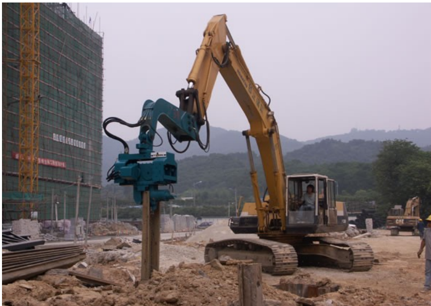
Figure 1.9: Pile vibratory technique. ( http://piling-equipment.com )
