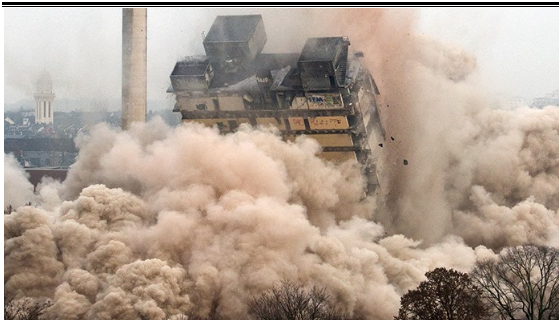
Figure 1.12: Demolition for a building, Frankfurt, Germany. ( www.rt.com/news/demolition-explosion-frankfurt-skyscraper-541 )
