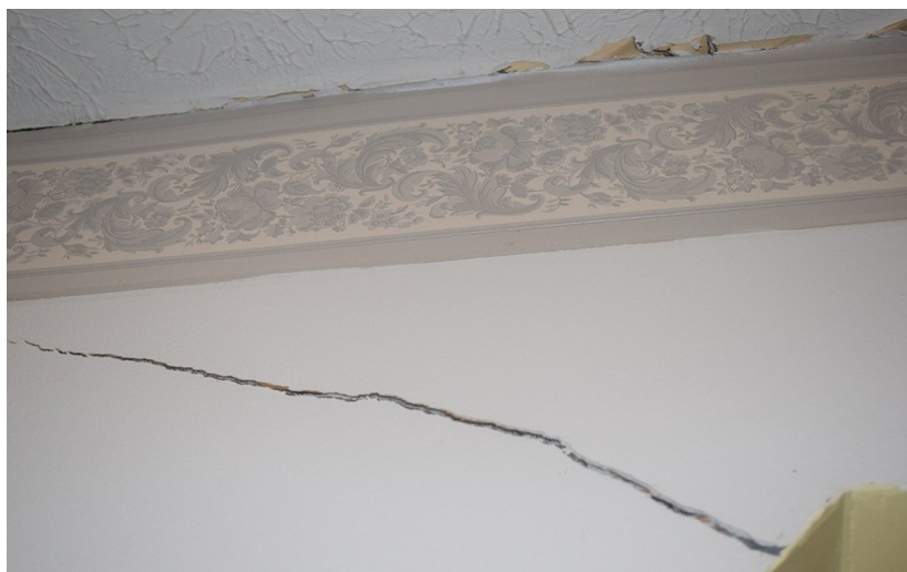
Figure 5.4: Sign of damage from the blasting, photo by Molly Moore, West Virginia USA. ( http://appvoices.org/2016/02/18/blasting-homeowners-property-damage-coal/ ).
