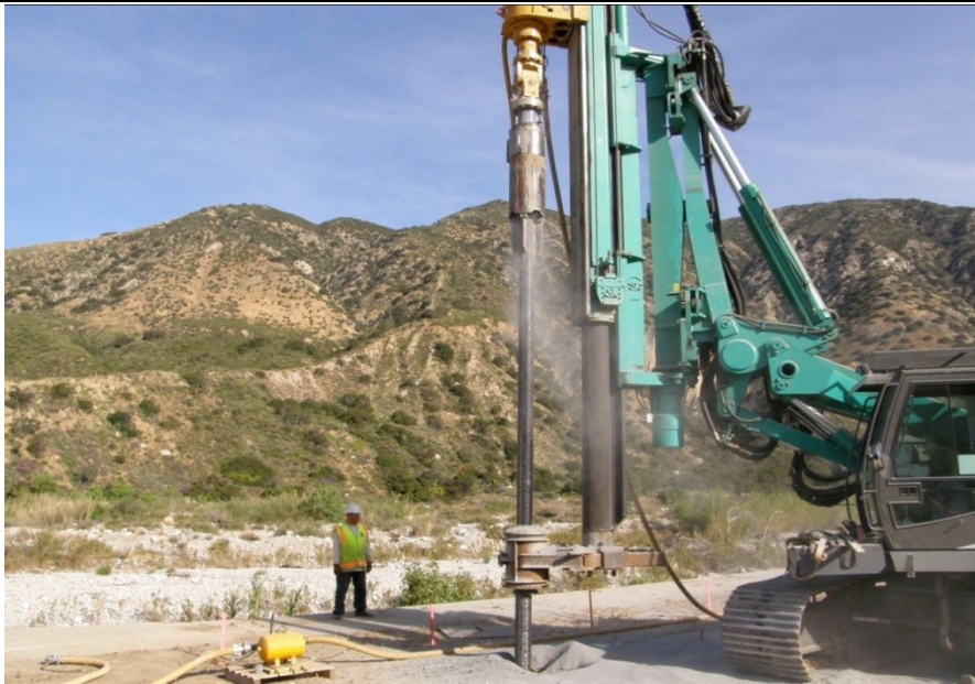
Figure 1.8: Pile driving technique hammer weight, ABI MOBILRAM, Lockhart Enterprises in Los Angeles, California.
