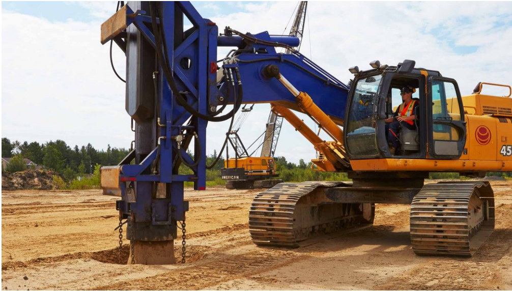
Figure 4.4: Rapid impact compaction machine, ( http://www.menardgroupusa.com )
