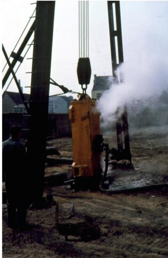
Figure 3.4: Double acting Steam hammer ( http://www.pilebuck.com )
