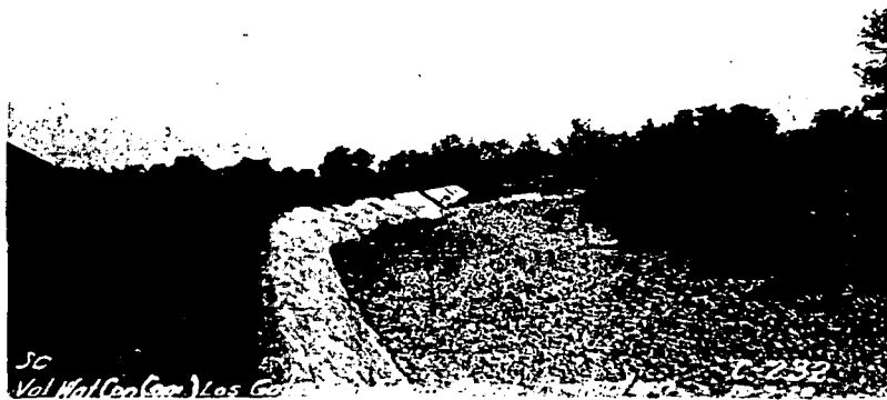
FIG. 2. Concrete Bank Protection at upper Duncan Ditch Headworks. Los Gatos Creek.
