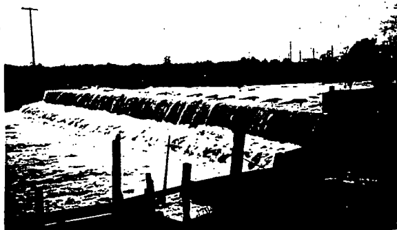
Waste water at Page Dam. Los Gatos Creek.
