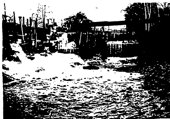
Waste Water Sorosis Dam-Campbell Creek.
