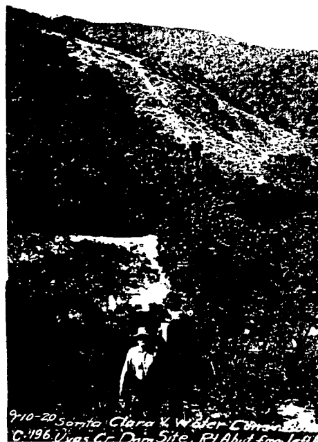
Uvas Dam Site-Right Abutment-
