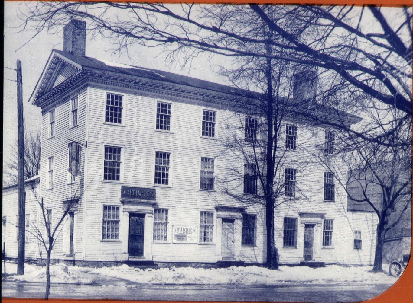
COLUMBIAN HOUSE, WATERVILLE, OHIO. Built 1828. On U. S. 24, facing the Maumee River, southwest of Toledo. An excellent example of New England Colonial, in wood, like the 1780 architecture of Massachusetts or Connecticut. The detail is unusually pure. Note the fluted pilasters and the thin bracketed cornice of the central doorway, the very elaborate eave and gable rake cornice, with frieze, dentals, bed-mold, modillions and crown. Built as a tavern. Stands essentially unchanged.
