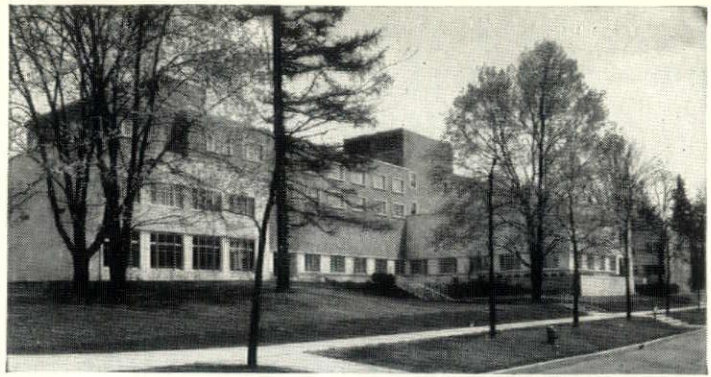
Statler Hall, Cornell University, Ithaca, N.Y. Holabird, Root & Burgee, architects, Chicago; Quackenbush Company, heating contractors, Buffalo.
