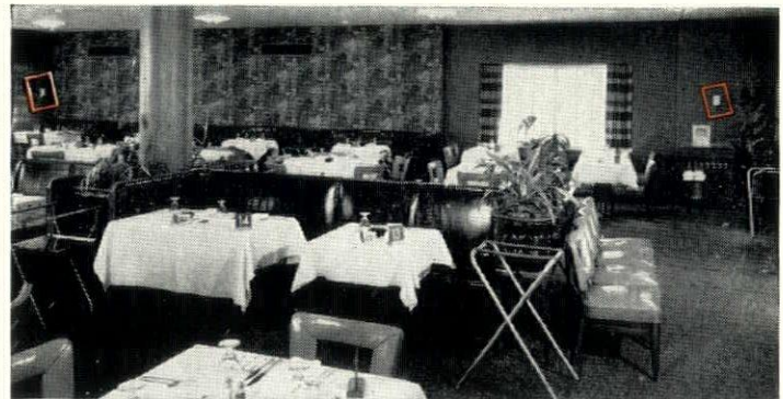
Johnson T-400 Room Thermostats operate valves on 105 convectors in public spaces such as the dining room.
