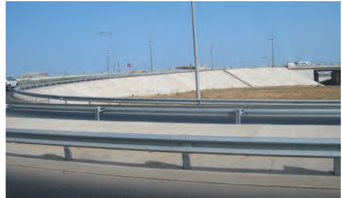
New traffic interchange section in Dakar
