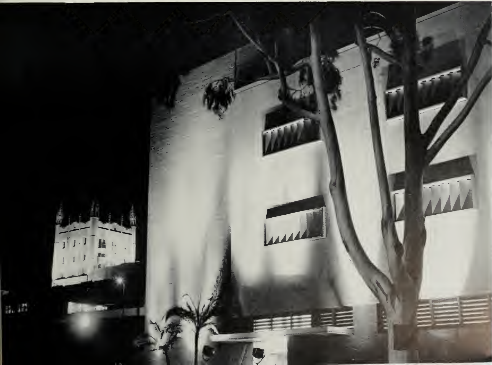
The Engineering Building is a hubbub of vital research and development activities both day and night.
